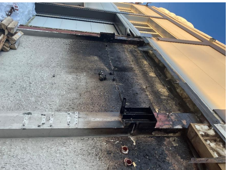
Wall 'B' Looking North with Garage Door
