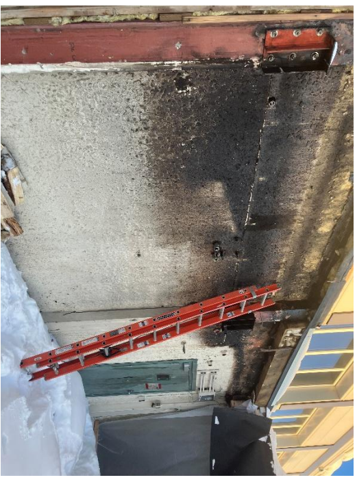
Wall 'B' and Wall 'A' Looking South
