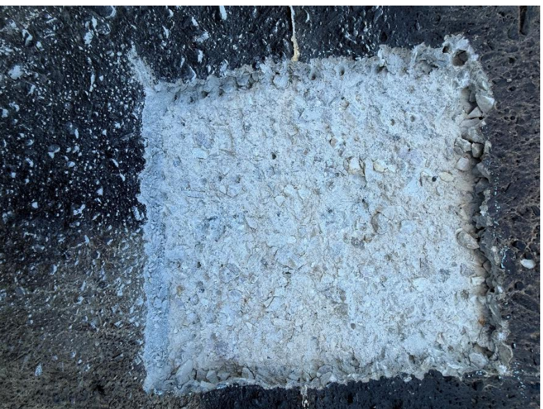
Test Patch – Wall 'B'
