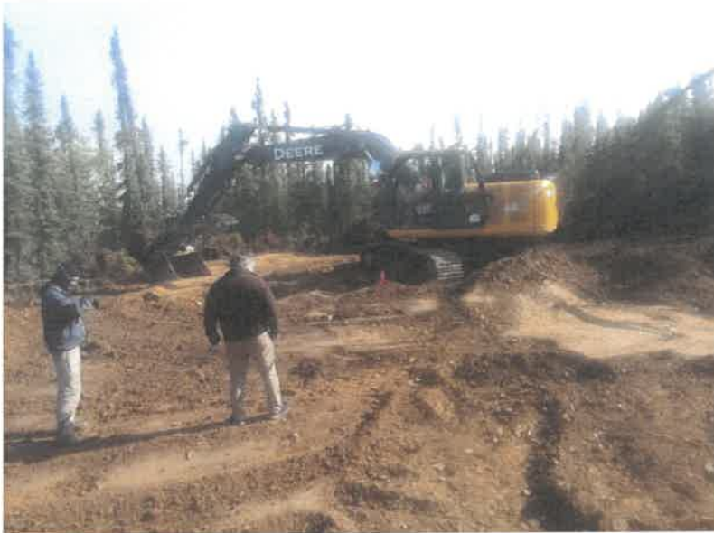
Figure 5: A drill pad from 2020 drill program on the Amanita claim block representative of the type of pad construction planned for the 2026-2028 drill program.
