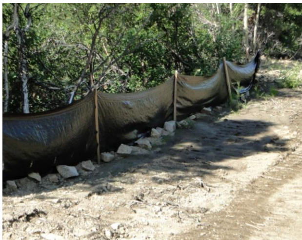
Examples of best management practices. Silt fence (left), elongated sediment ponds (right)
