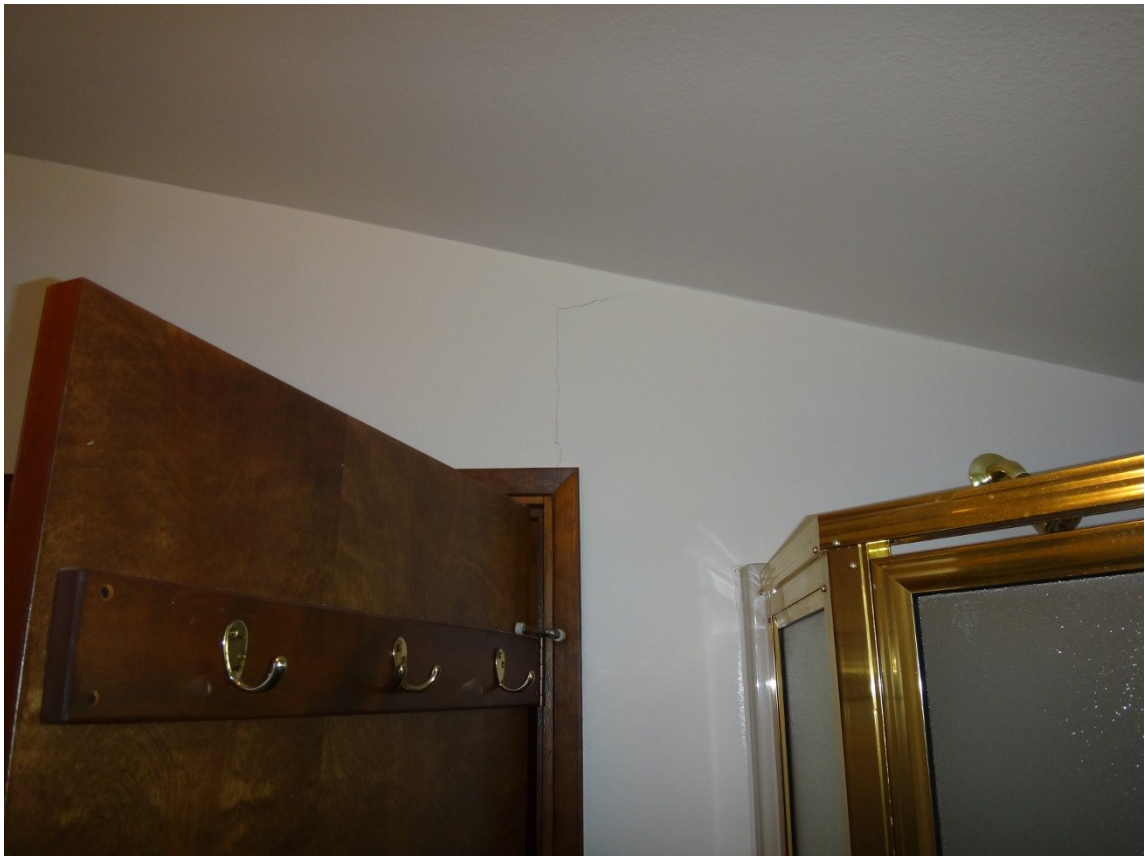
Wall Crack
