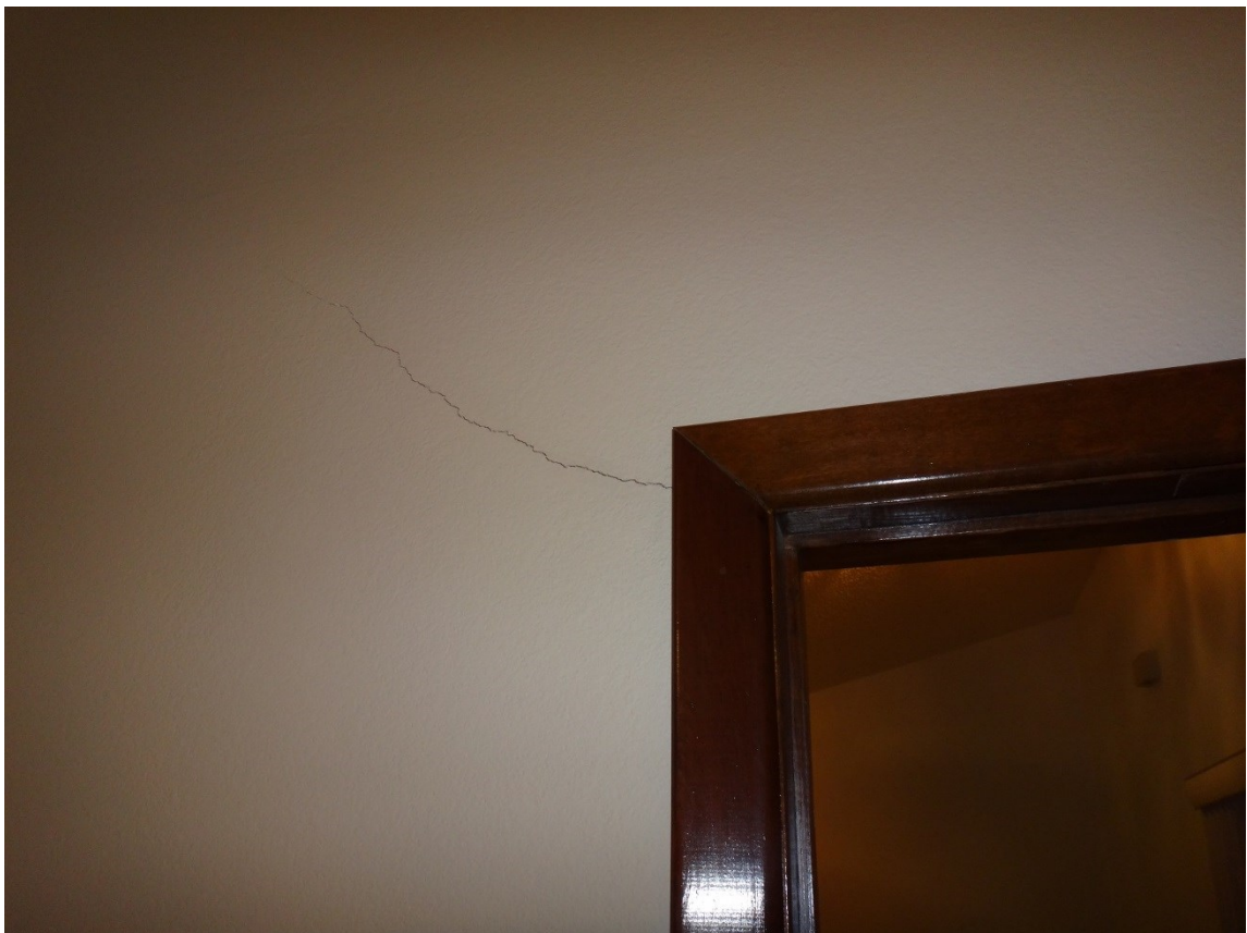
Wall Crack
