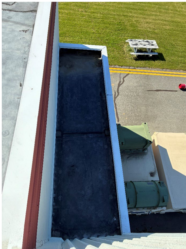
Southwest Lower Roof Area Photo
