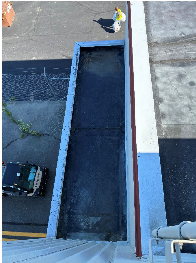
Northwest Lower Roof Area Photo
