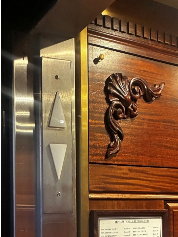
Elevator Car Interior Direction Indicators
