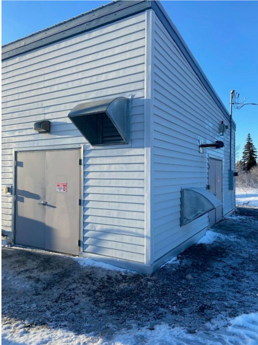
Figure 1 Manokotak Heights Generator Building
