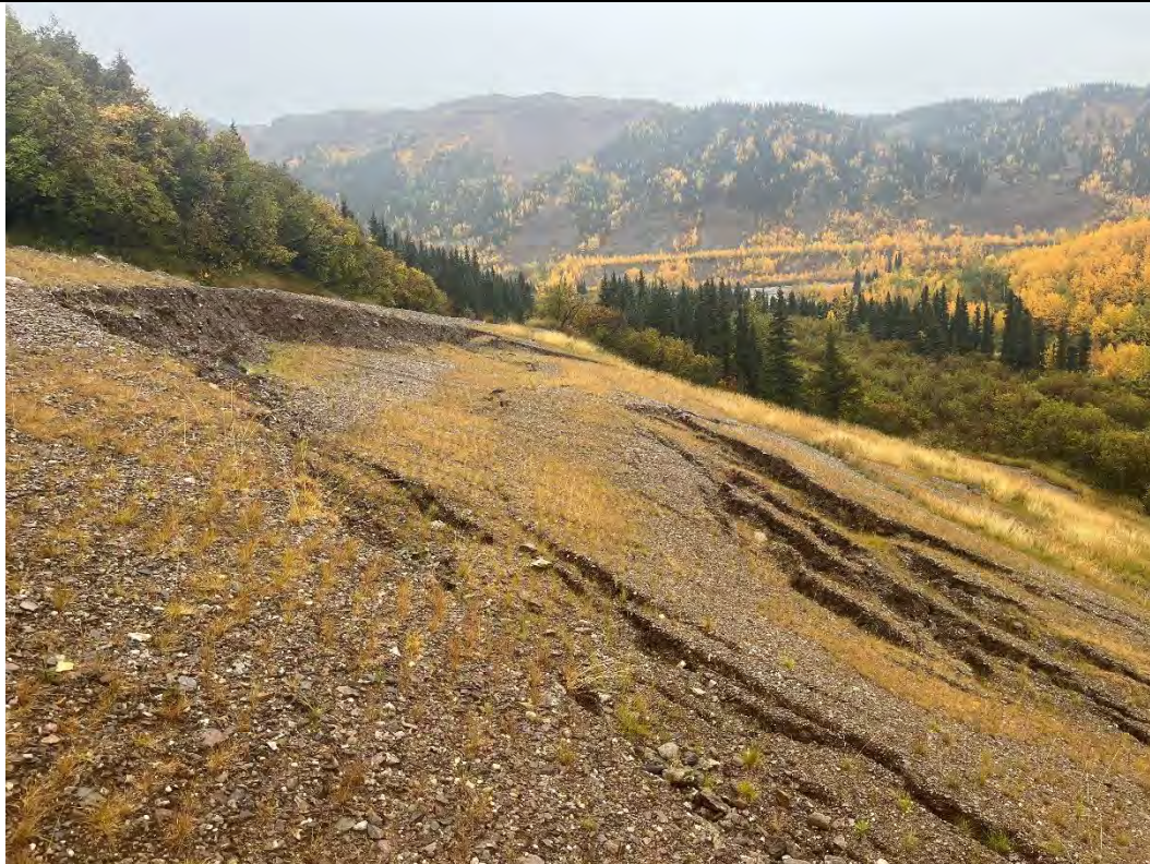
Photo 6. Unstable Slope – Site Visit – View Northwest
