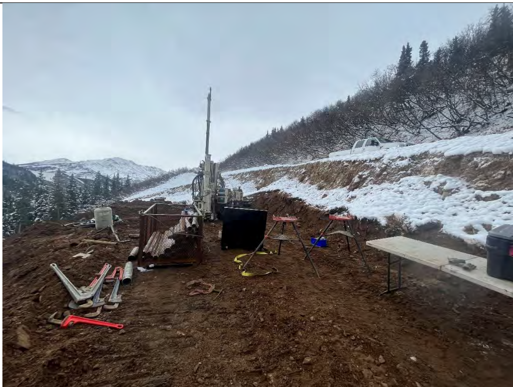
Photo 11. Slope Investigation – Test Boring 1 Location
