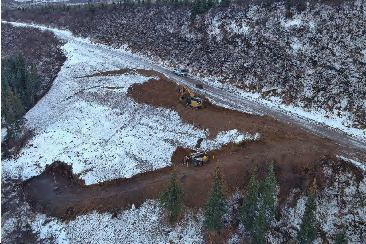
Photo 9. Slope Investigation – Aerial View South with Tests Boring Locations Shown
