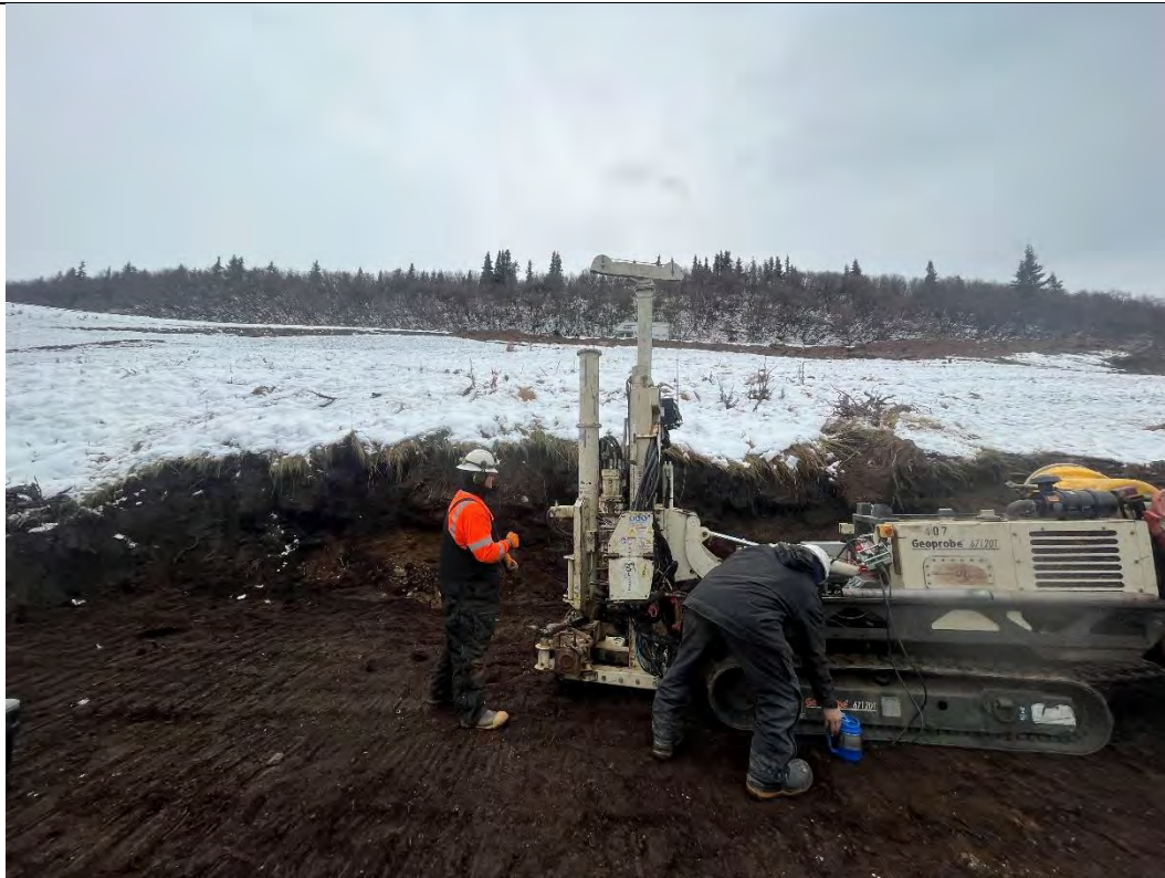
Photo 13. Slope Investigation – Test Boring 2 Location at Toe of Fill
