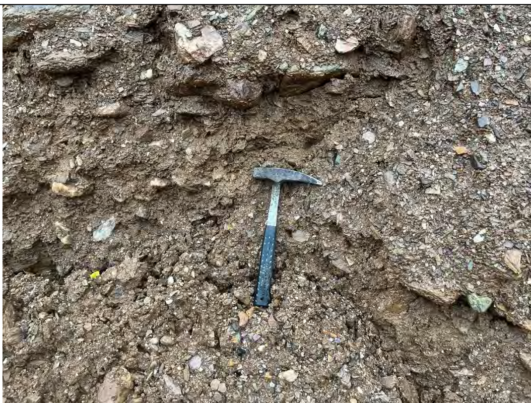
Photo 8. Unstable Slope – Material Exposed in Scarp
