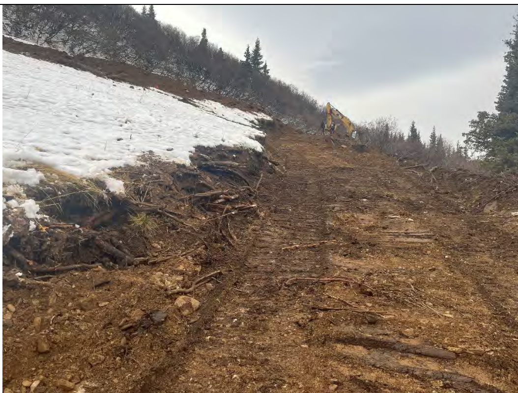
Photo 12. Slope Investigation – View Northwest of Access Path to Test Boring 2
