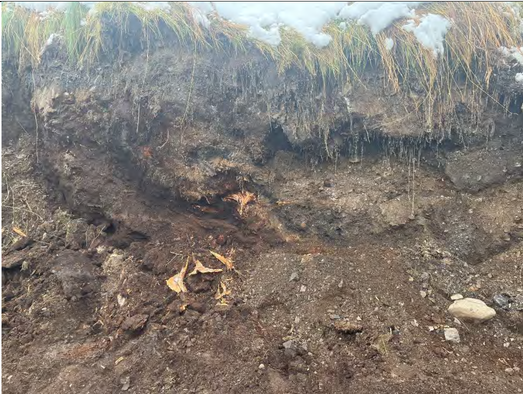
Photo 17. Slope Investigation – Photo #3 of Toe Material Exposed Upslope of Test Boring 2
