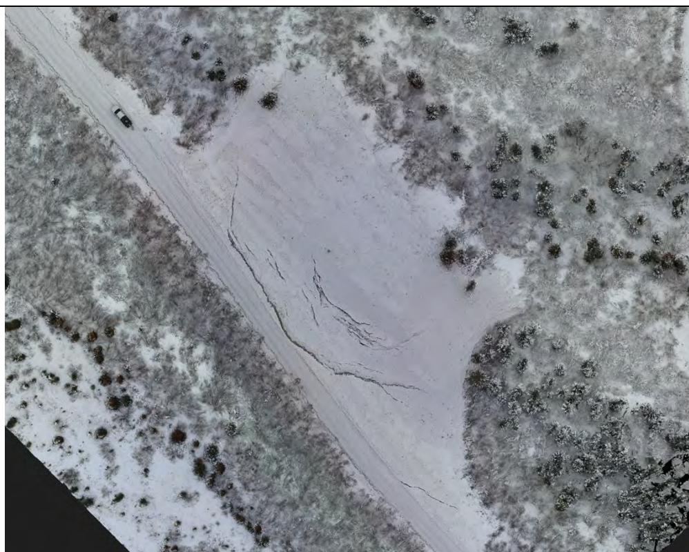
Photo 4. Unstable Slope – Aerial Nadir View
