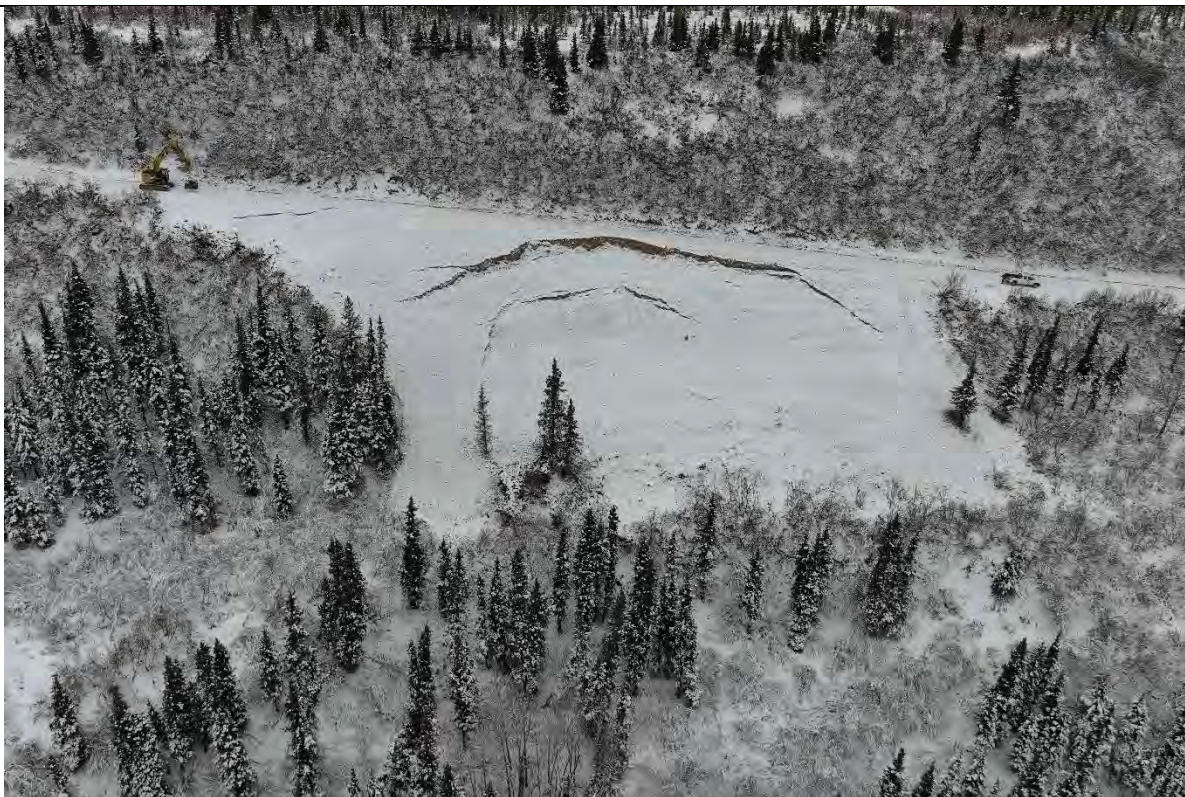
Photo 3. Unstable Slope – Aerial View West
