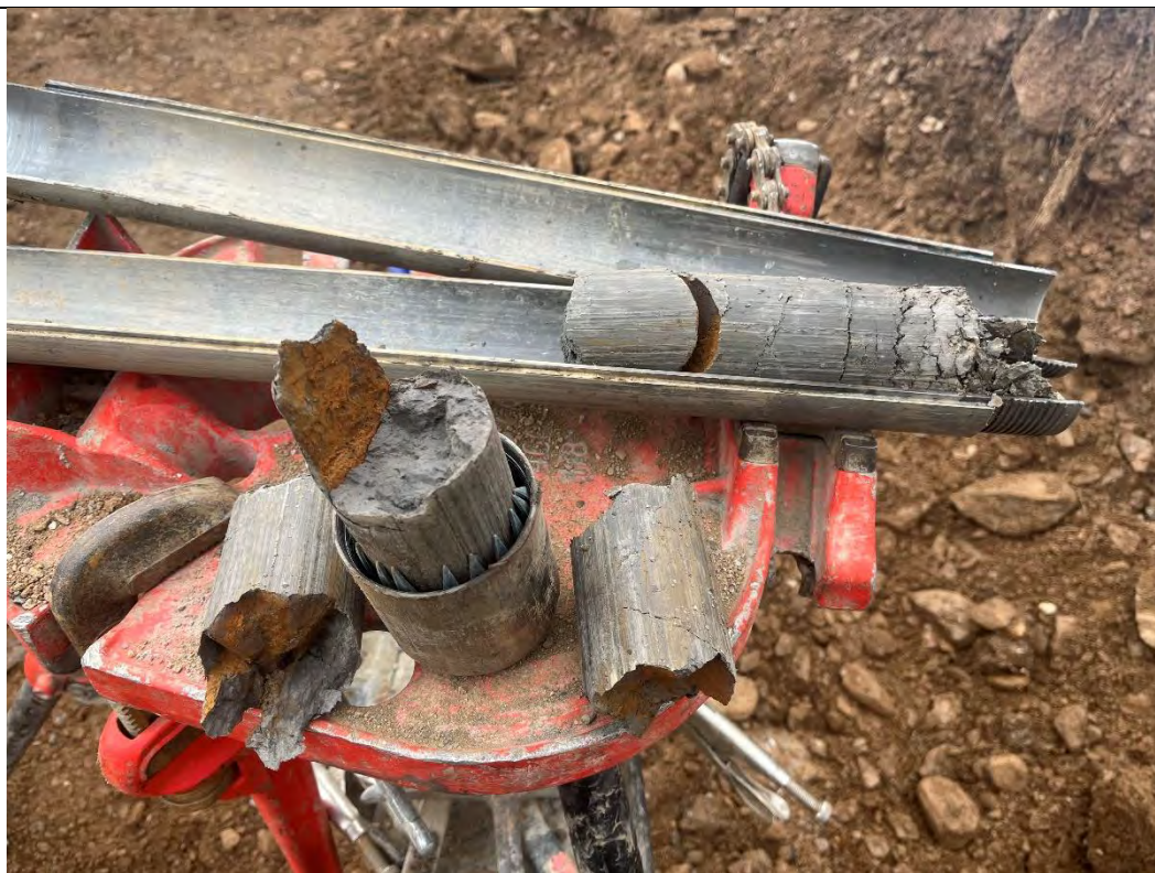
Photo 17. Slope Investigation – Claystone Material with Planar and Curved Discontinuities
