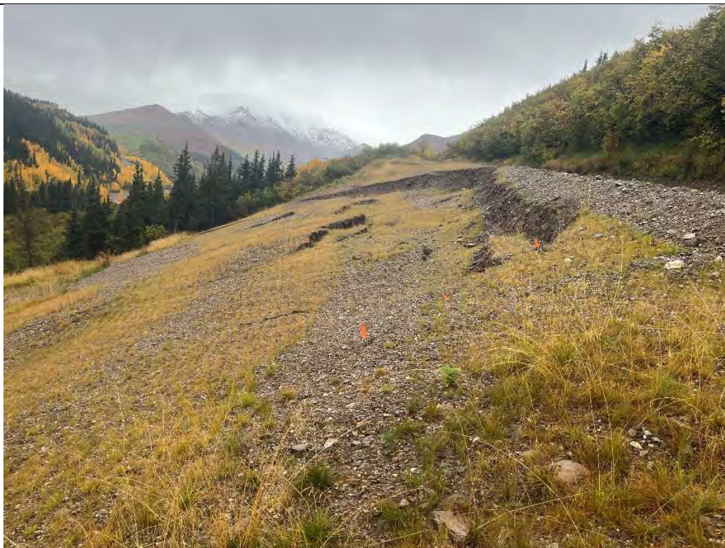
Photo 5. Unstable Slope – Site Visit – View Southeast
