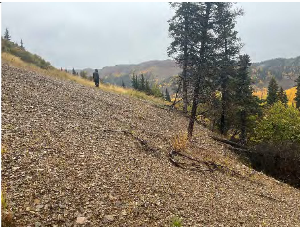
Photo 7. Unstable Slope – Site Visit – View Northwest from Southeast Toe
