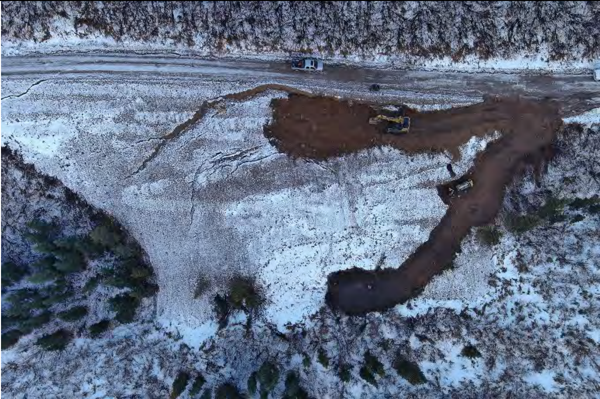
Photo 10. Slope Investigation – Nadir Aerial View with Tests Boring Locations Shown
