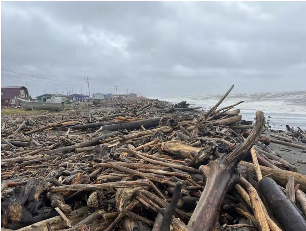
Figure 10. Shaktoolik's berm destroyed in the storm
