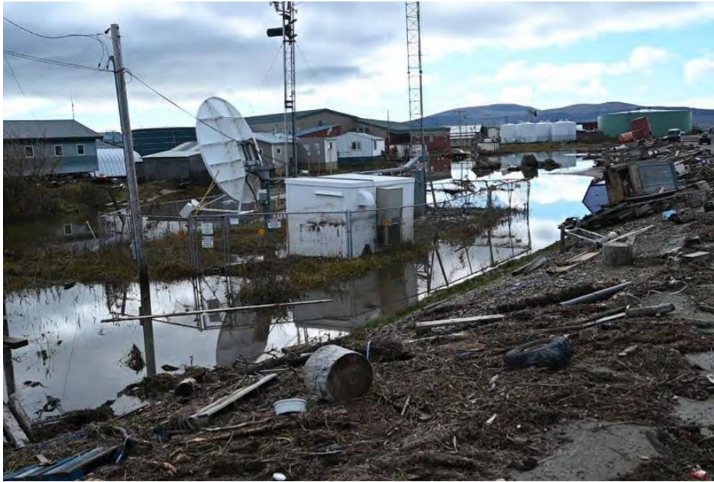
Figure 12. Storm Debris in Golovin on September 20, 2022
