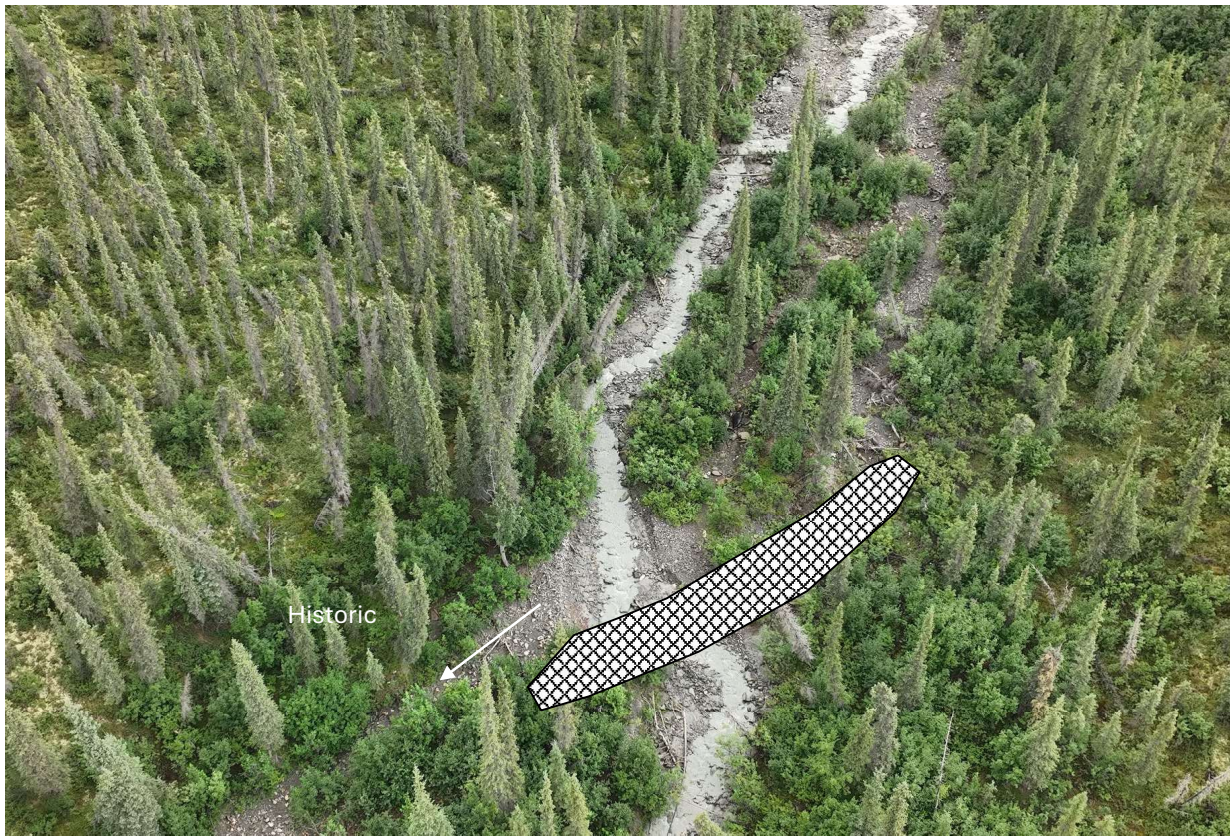
Dike Layout – spanning the dike across the entire channel will capture any flow that enters the secondary channel.
