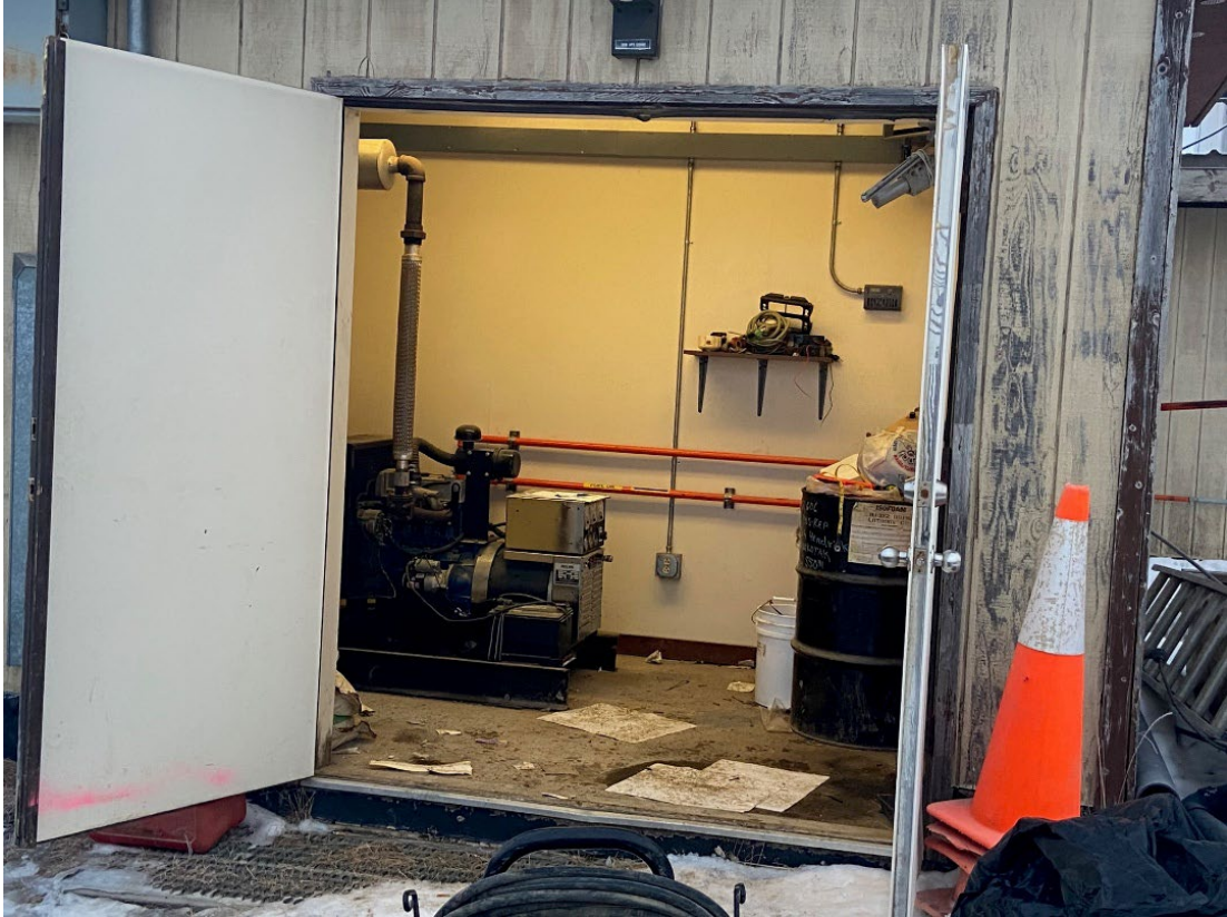
Figure 4 Old Village Generator Building
