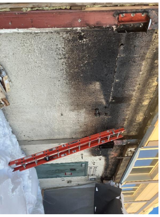
Wall 'B' and Wall 'A' Looking South
