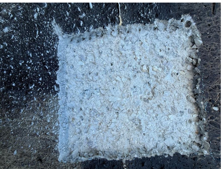
Test Patch – Wall 'B'
