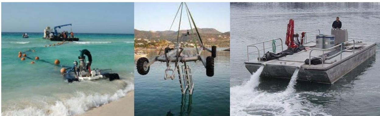
Figure 24: Jetting sled and support barge for the shore end operations.
