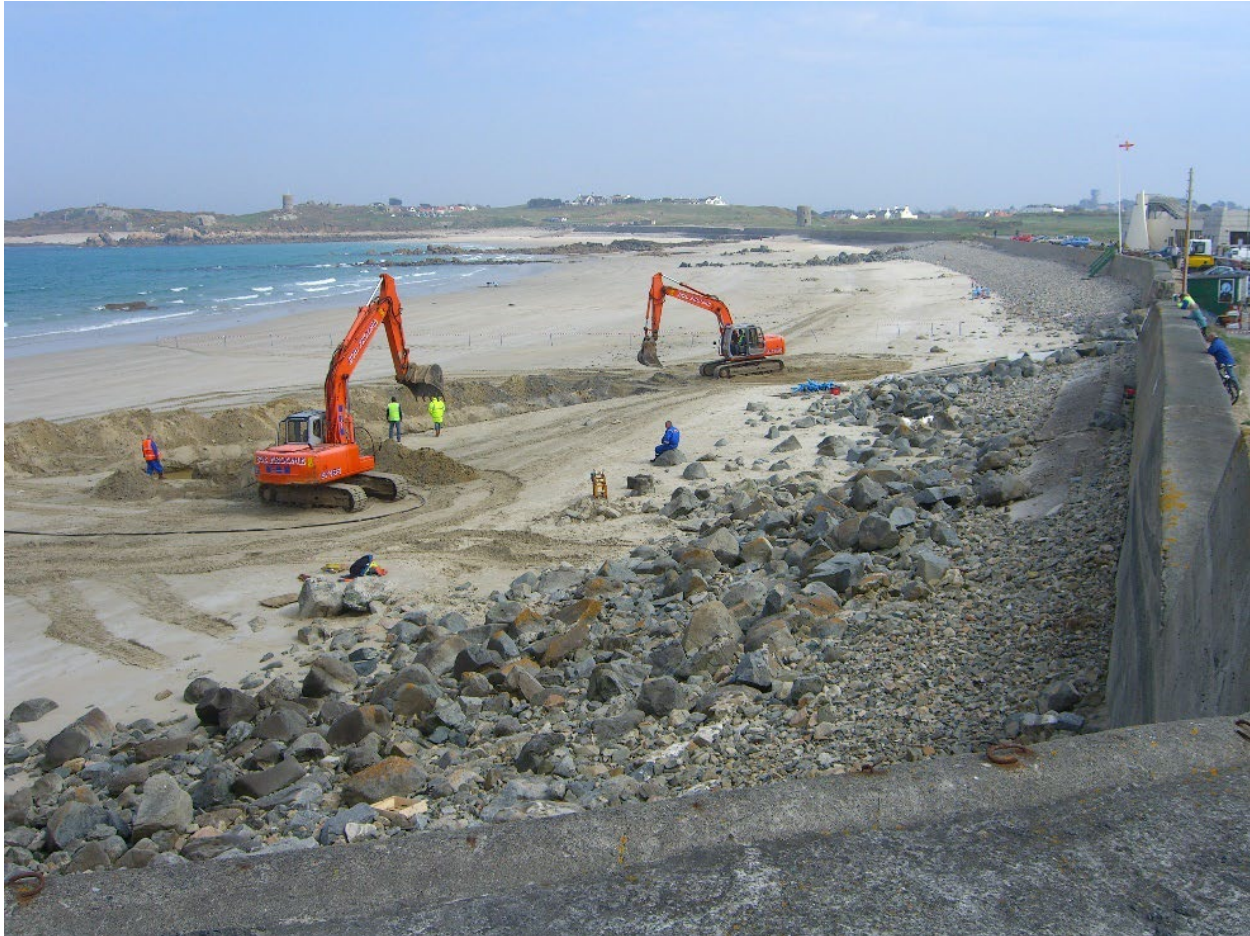
Figure 23: Example trench digging on beach.
