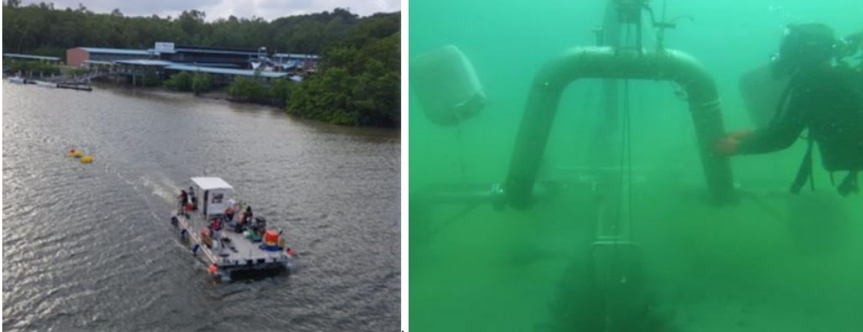
Figure 25: Support barge and jetting sled for the shore end operation.
