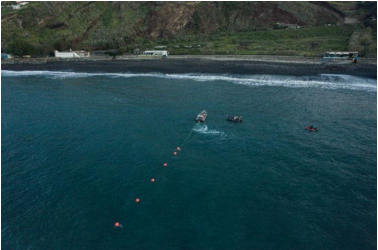
Figure 17: Workboat delivering a cable to a duct exit.
