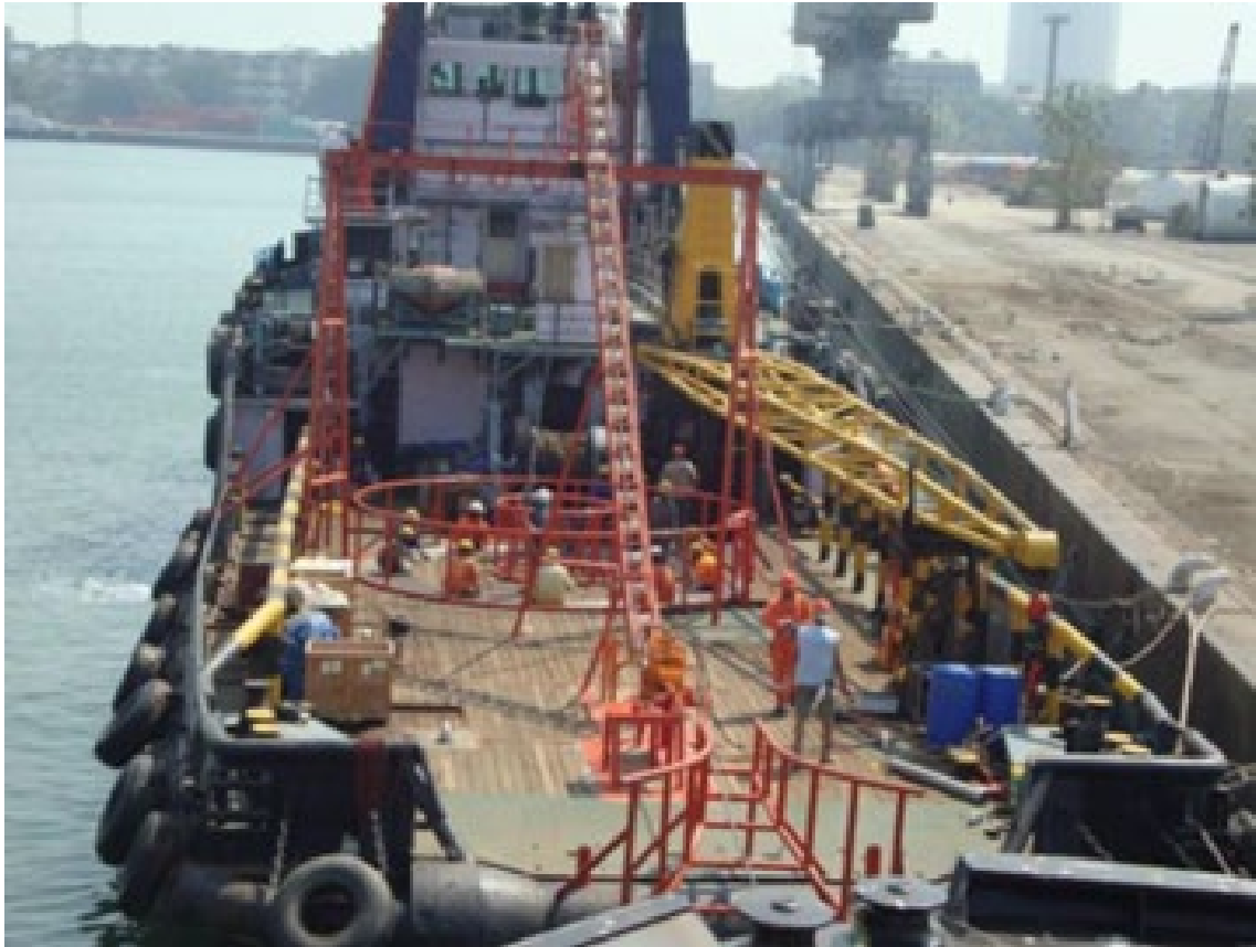
Figure 16: Example shore end installation vessel
