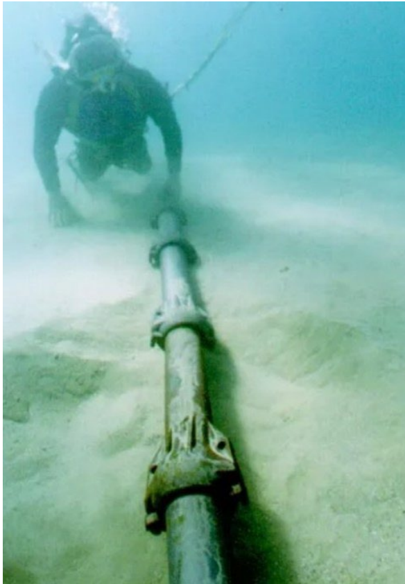
Figure 27: Articulated pipe installation.
