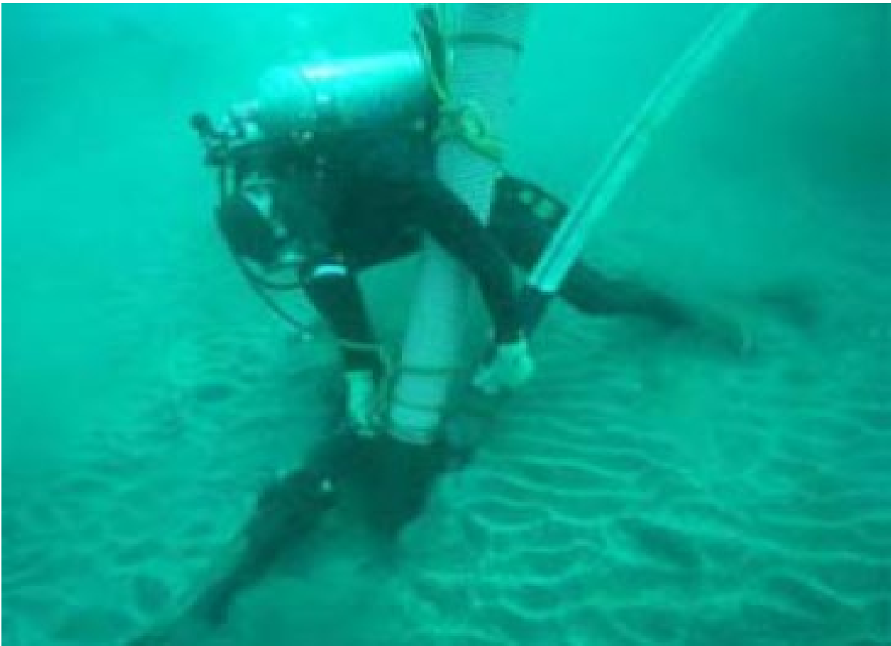
Figure 26: Diver assisted hand jetting via an air-lift.
