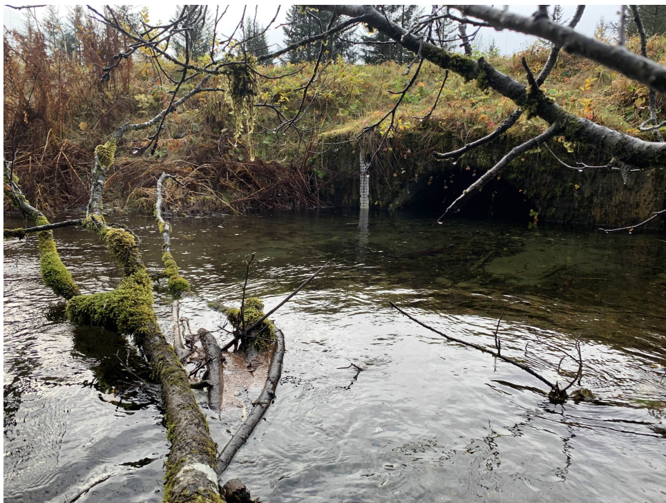
Photo 8: Cannon Beach Rd stream culvert crossing Airport Rd, facing south.
