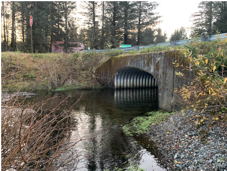
Photo 12: Yakutat Airport stream culvert under Airport Access Rd, facing west.
