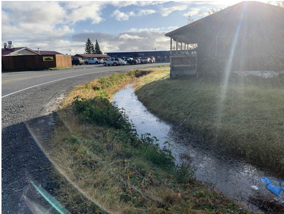
Photo 11: Yakutat Airport Trib 4 where road curves to Alaska Airlines terminal building, facing northeast.
