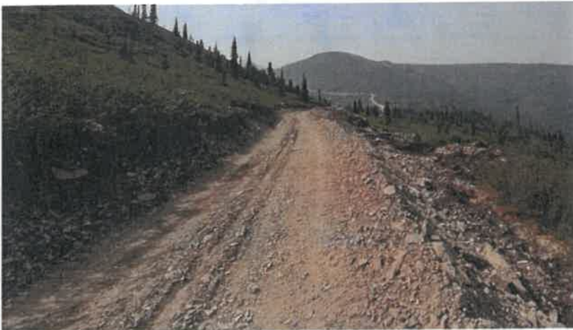
Figure 7. Typical trail construction.
