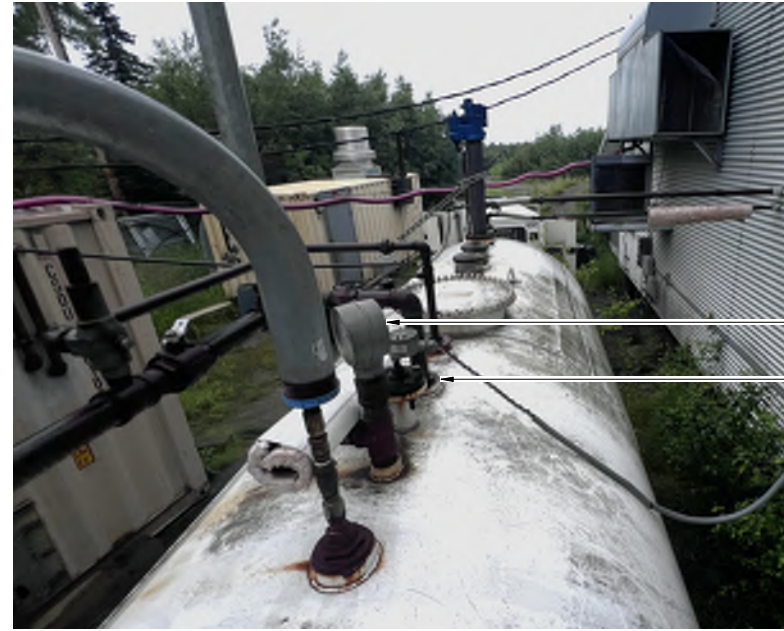
2 SCHOOL TANK APPURTENANCES PHOTO SCALE: NTS
