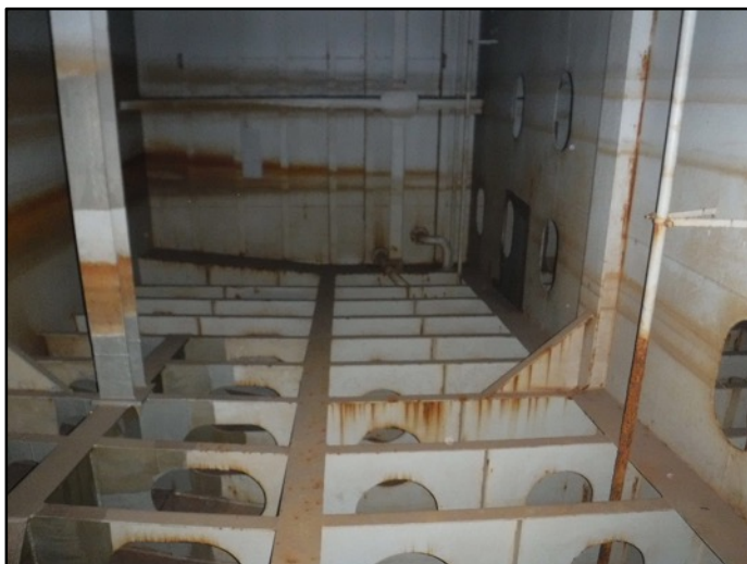
Photo 53: Existing Coating System in No. 11 Center Line Ballast
