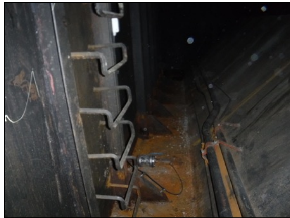
Photo 25: No. 5 Starboard Void
