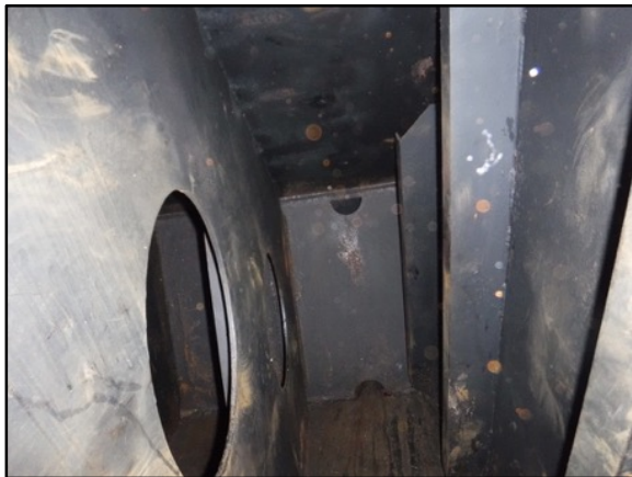
Photo 27: No. 5 Port Wing Void
