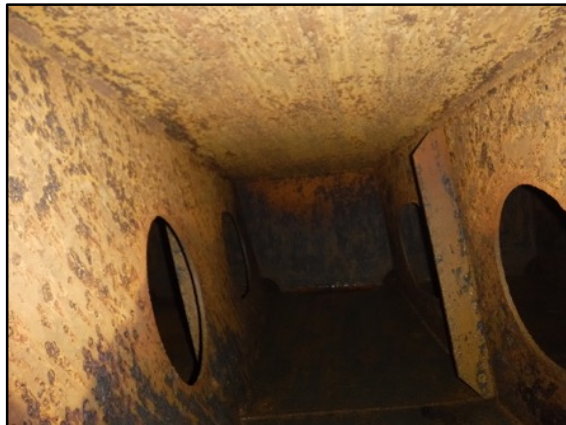
Photo 21: No. 4 Starboard Wing Ballast
