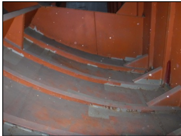
Photo 39: No. 10 Starboard Void
