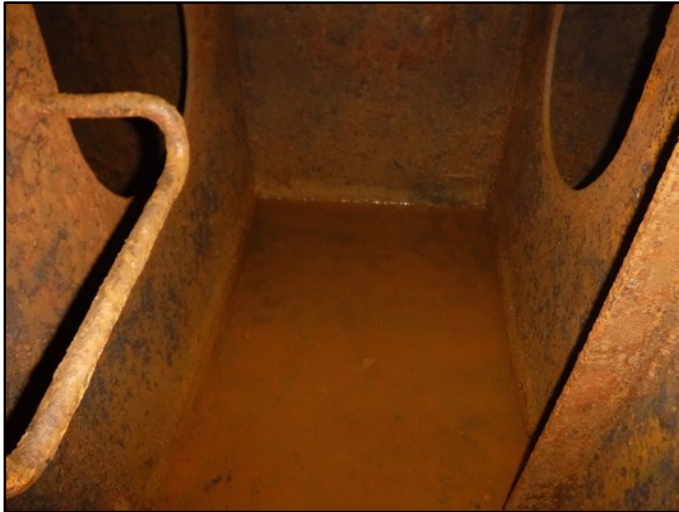
Photo 22: No. 4 Center Line Double Bottom Ballast
