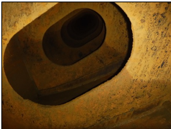
Photo 32: No. 8 Port Wing Ballast
