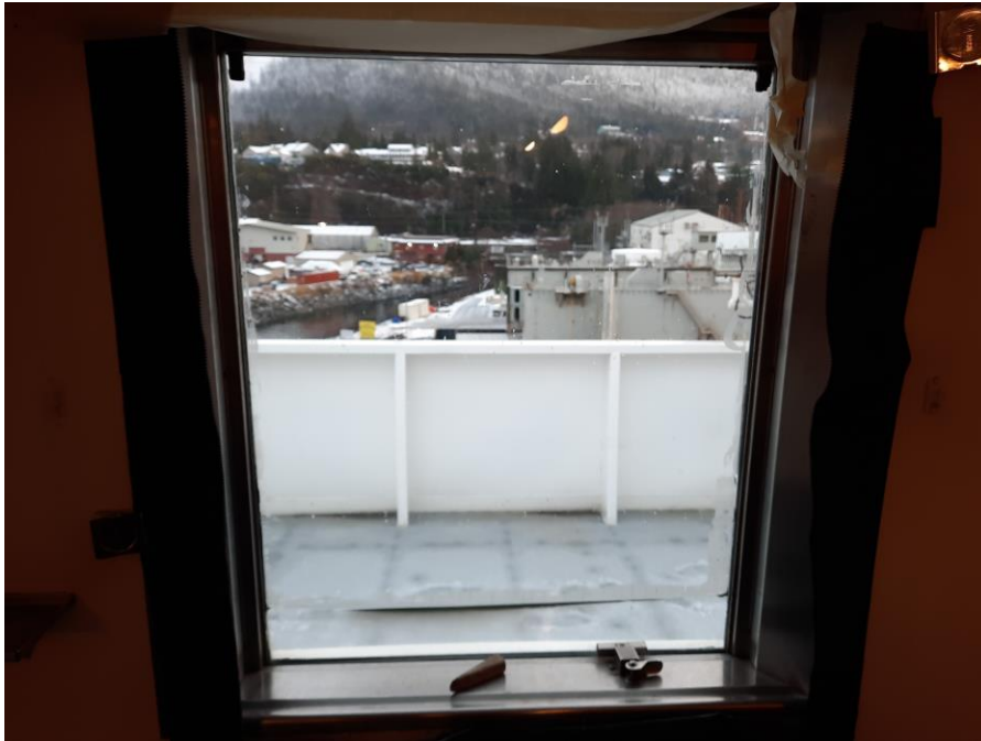
Figure 20 Single pane window in 2nd Mate Stateroom
