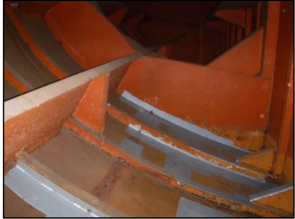
Photo 47: No. 11 Starboard Void
