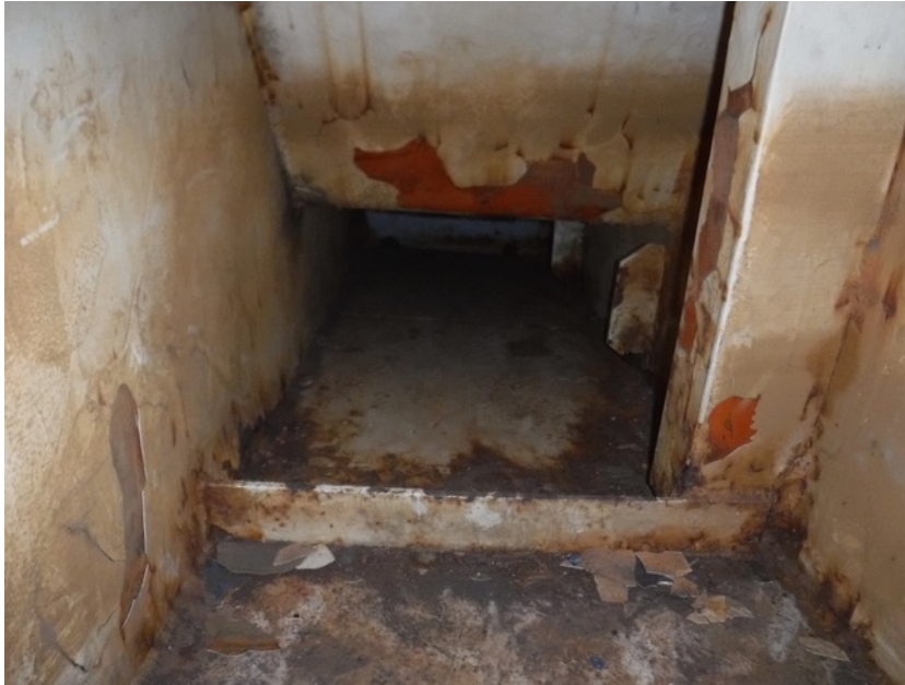
Photo 41: Minor Corrosion in Lower Section of No. 10 Port Void
