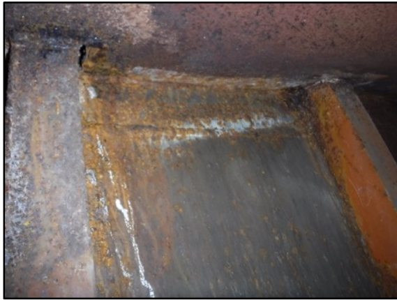
Photos 16 & 17: Corrosion on Skin Plate Above Starboard Wing Ballast
