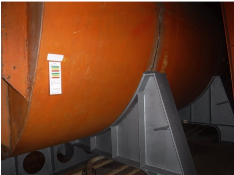
Photo 15: Existing Coating System in No. 4 Void
