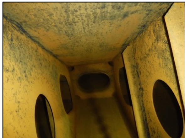
Photo 33: No. 8 Starboard Wing Ballast
