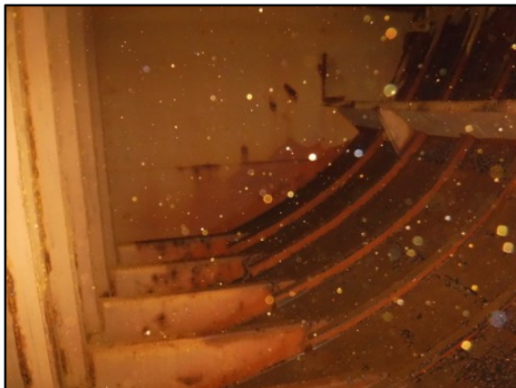
Photo 34: No. 9 Port Wing Void
