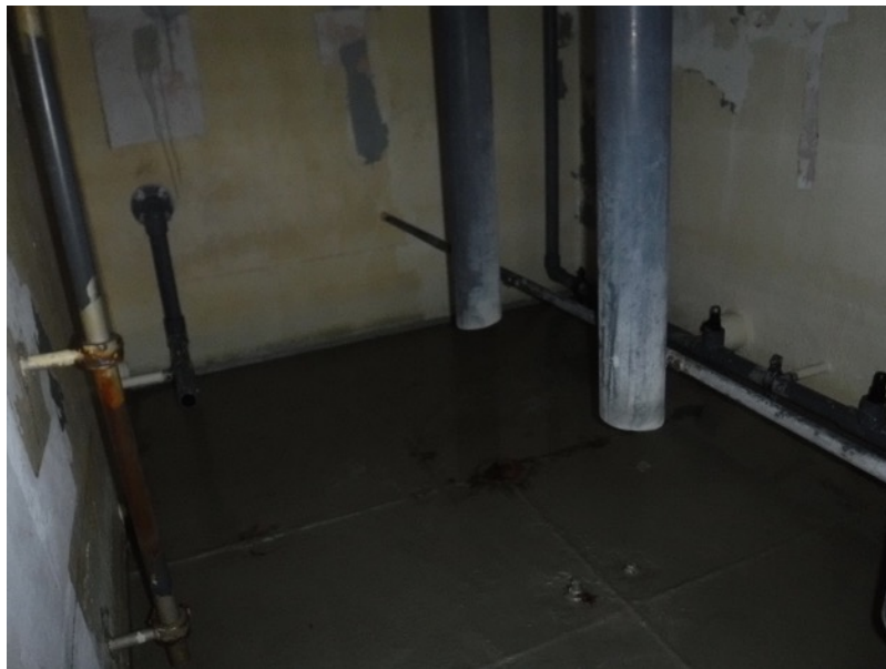
Photo 30: Existing Coatings in V-1 Sewage Tank
