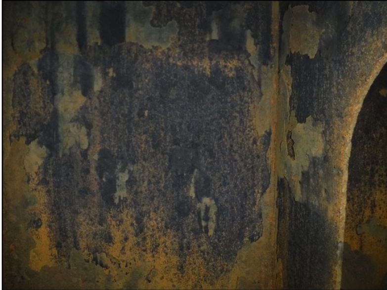
Photo 37: Coating Delamination Spots
