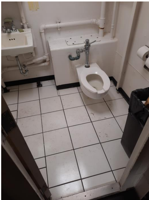
Figure 21 New deck covering in Engineer's Head
