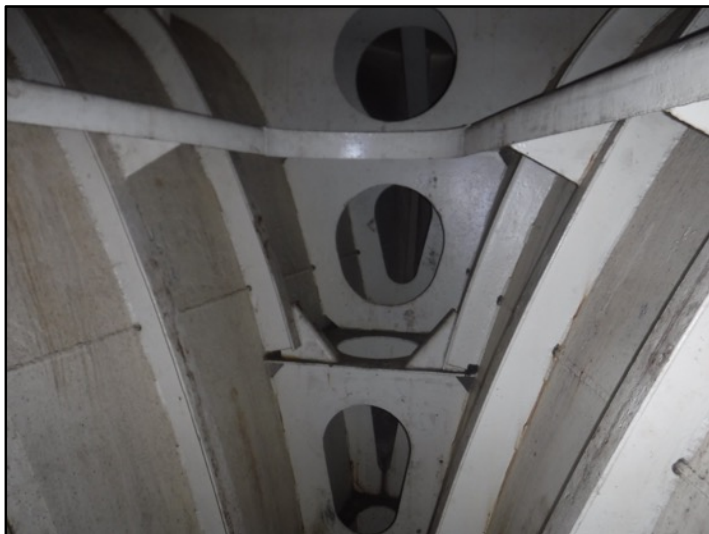
Photo 1: Existing Coating System in the Forepeak
