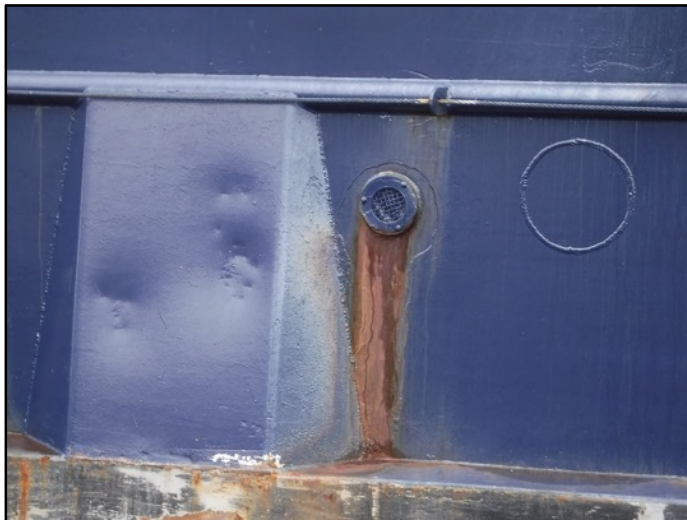
Photo 65: Rust Bleed Under Vents & Drains
