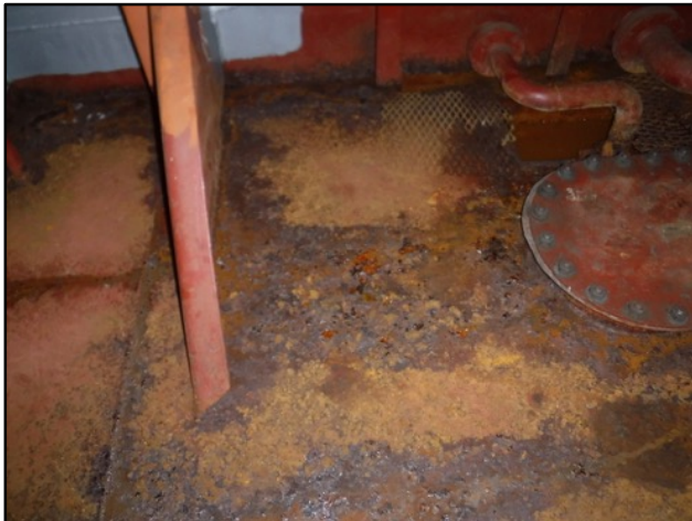
Photo 11: Corrosion on Deck near Aft Bulkhead
