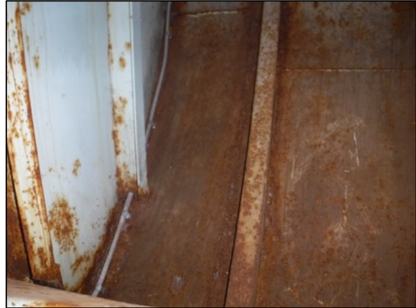
Photos 48 & 49: Corrosion on Skin Plate in Forward Section of Both Voids
