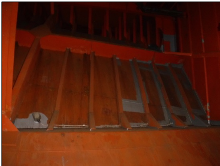
Photo 9: Existing Coating System in No. 3 Void
