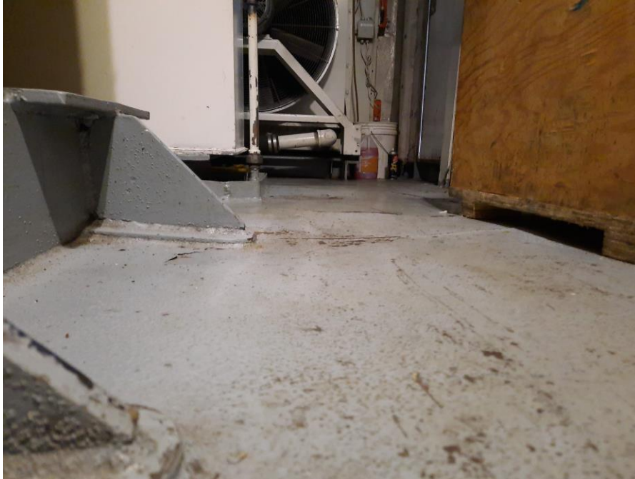
Figure 28 Emergency Generator Room deck coatings
