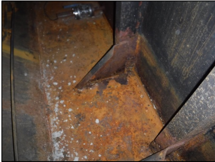
Photo 26: Corrosion near Centerline Bulkhead in No. 5 Starboard Void
