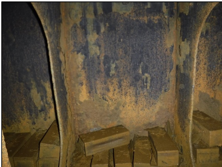
Photo 36: Existing Coating System in No. 9 Double Bottom Ballast
