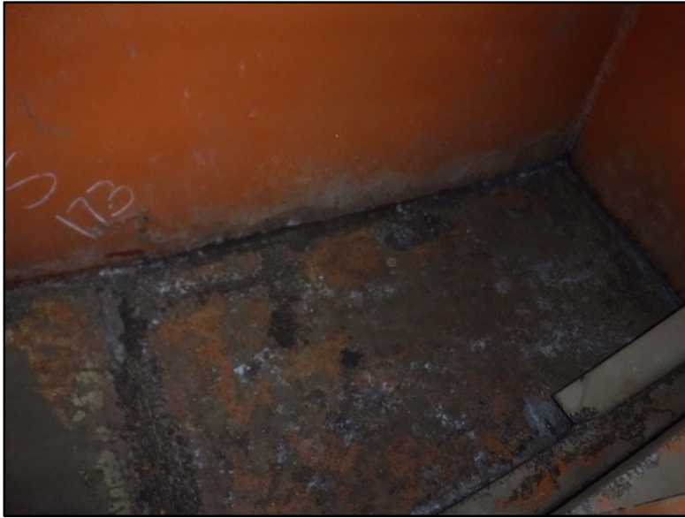
Photo 52: Corrosion on Deck of Cross Flood
