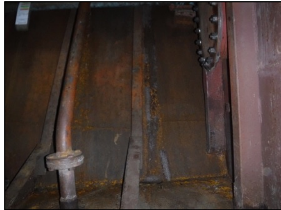
Photos 16 & 17: Corrosion on Skin Plate Above Starboard Wing Ballast
