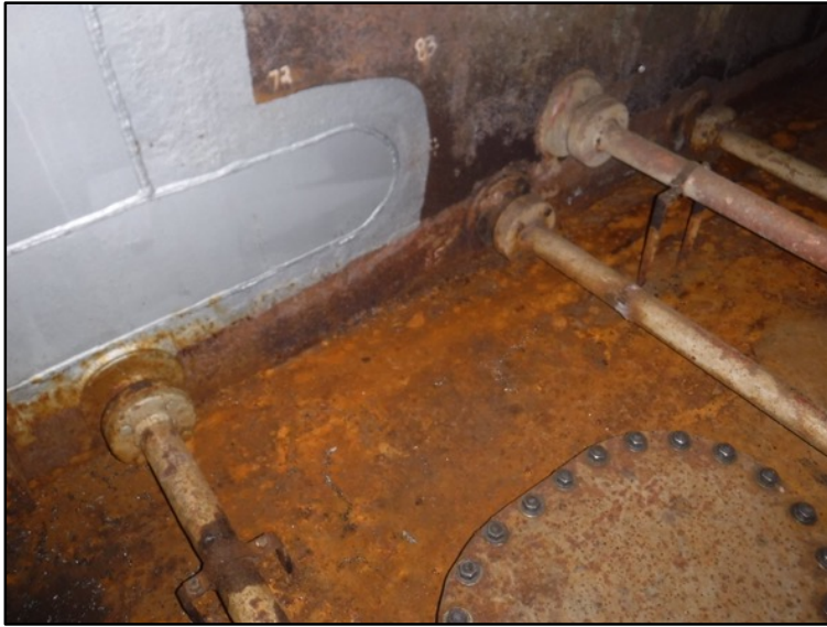
Photo 19: Corrosion on Deck Near Forward Bulkhead
