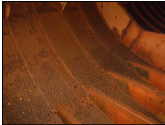
Photo 35: No. 9 Starboard Wing Void
