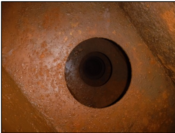
Photo 12: Port Wing Ballast
