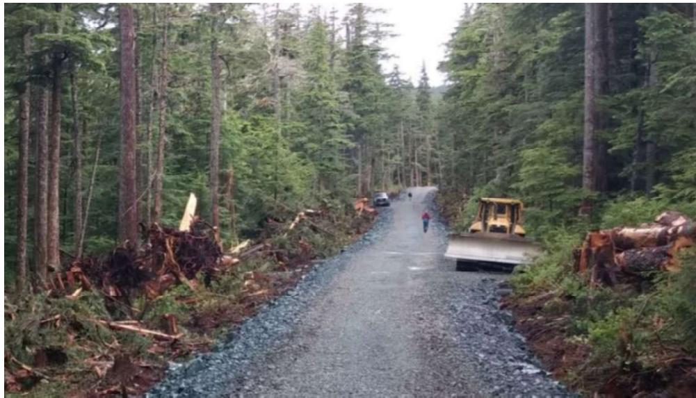
Along the roadway, two 1-acre pads will be developed to serve as equipment laydown & helipad areas, both consisting of a 2-3ft bed of compacted shot rock.
