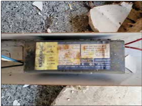
PHOTO 8: LOT 3 - TYPICAL ASSUMED PCB CONTAINING BALLAST.
