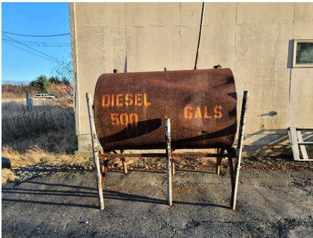
Photo 14: Example of a 500-gallon diesel fuel tank located on Lot 5A. The tank is in poor condition and should not be reused.
