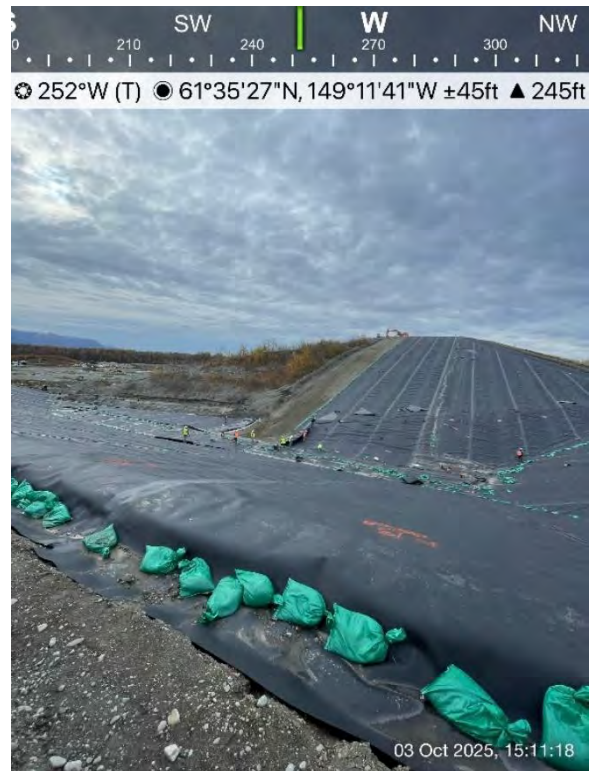
Figure 28: 10/05/25 – West Side of Existing Cell 2B GCL Exposed and Sprinkled with Granular Bentonite
