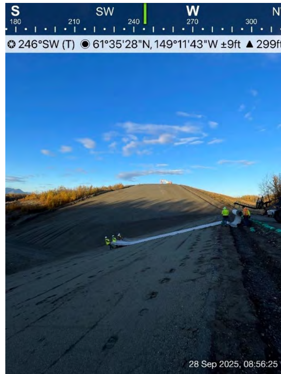
Figure 4: 09/28/25 – GCL Panel Overlapped a Min. of 12 Inches and Sprinkled with Granular Bentonite Prior to Heat Tack
