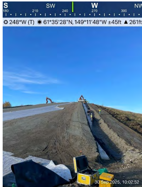
Figure 14: 09/30/25 - Cell 4 Expansion GCL Placement Day 3
