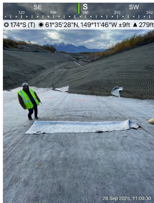
Figure 4: 09/28/25 – GCL Panel Overlapped a Min. of 12 Inches and Sprinkled with Granular Bentonite Prior to Heat Tack
