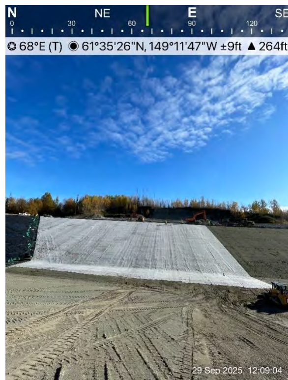
Figure 10: 09/29/25 - Cell 4 Expansion GCL Placement Day 2
