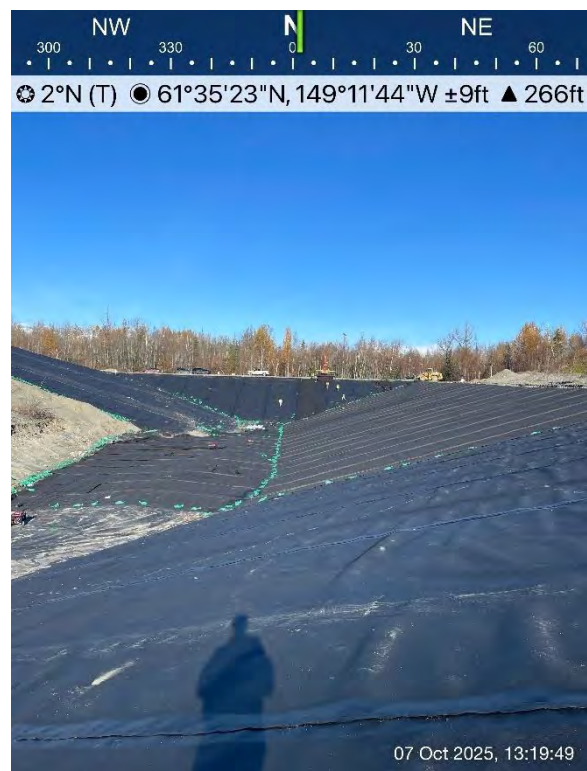
Figure 34: 10/07/25 - Cell 4 Expansion Geotextile Cushion Deployment with Spreader Bar
