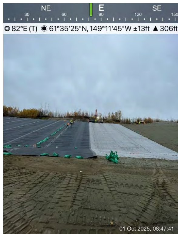
Figure 18: 10/01/25 - Cell 4 Expansion GCL Placement Day 4
