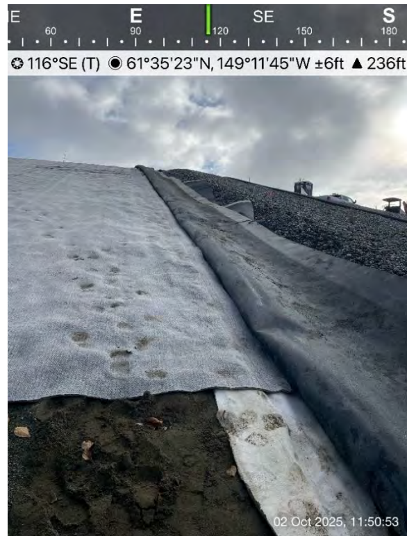
Figure 22: 10/02/25 - Cell 4 Expansion GCL Overlapped with Existing Cell 2B GCL
