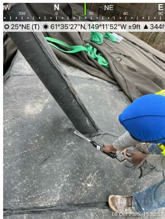
Figure 38: 10/08/25 – Non-Destructive Spark Testing of Pipe Boot
