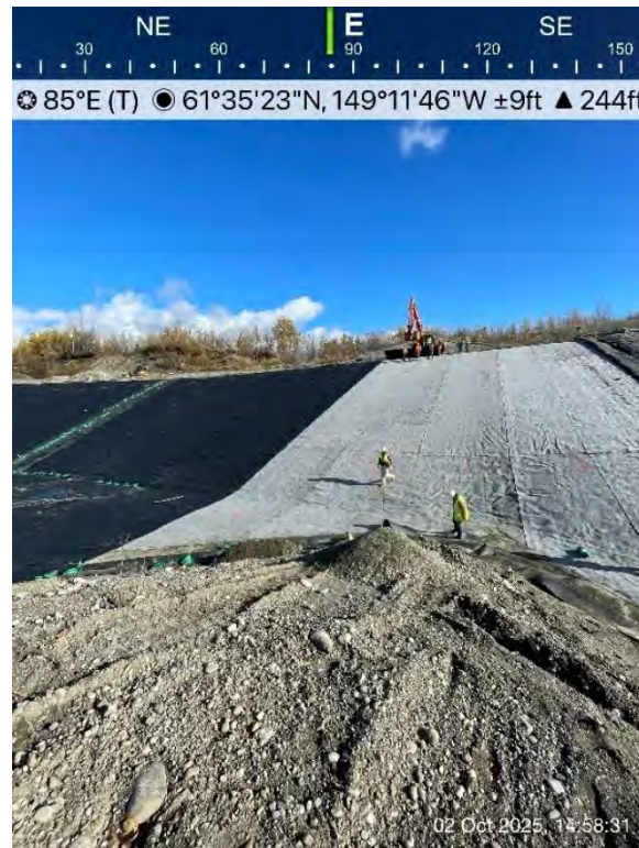
Figure 24: 10/02/25 - Cell 4 Expansion GCL Placement Day 5
