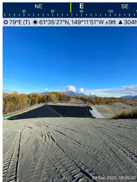
Figure 12: 09/29/25 - Cell 4 Expansion HDPE Geomembrane Liner Placement Day 2
