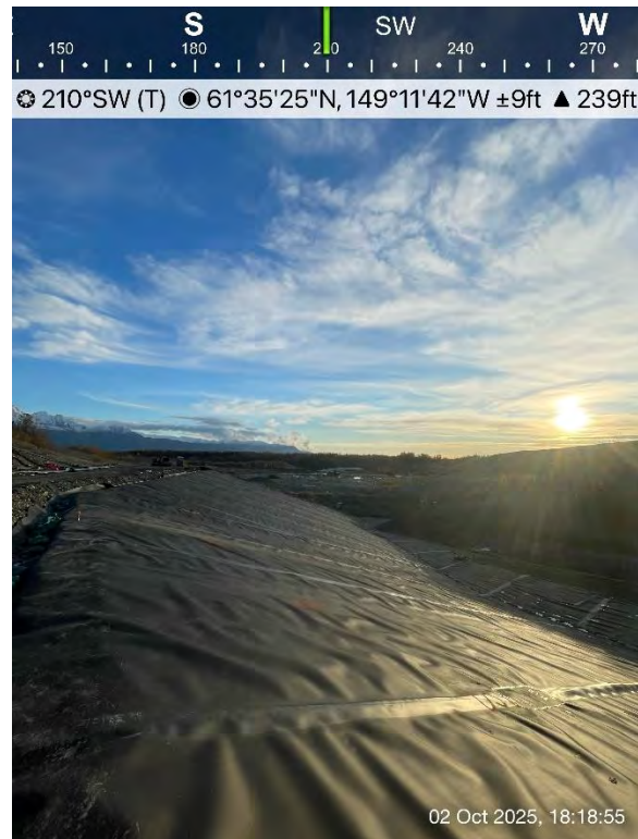
Figure 26: 10/03/25 - Cell 4 Expansion GCL Placement Day 6
