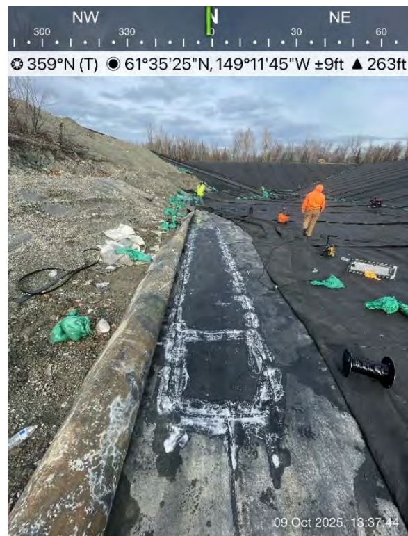
Figure 40:10/08/25 – Extrusion Patch of DS-20 and Bounding Samples
