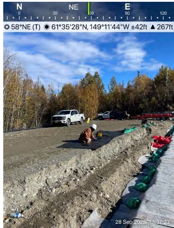
Figure 8: 09/28/25 - Cell 4 Expansion HDPE Geomembrane Liner Placement Day 1
