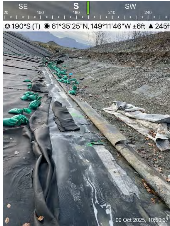
Figure 40:10/08/25 – Extrusion Patch of DS-20 and Bounding Samples
