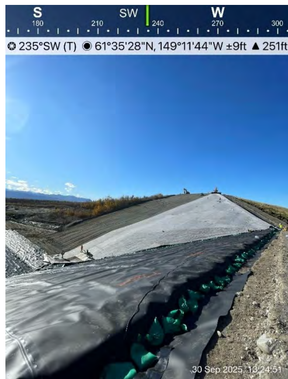
Figure 14: 09/30/25 - Cell 4 Expansion GCL Placement Day 3
