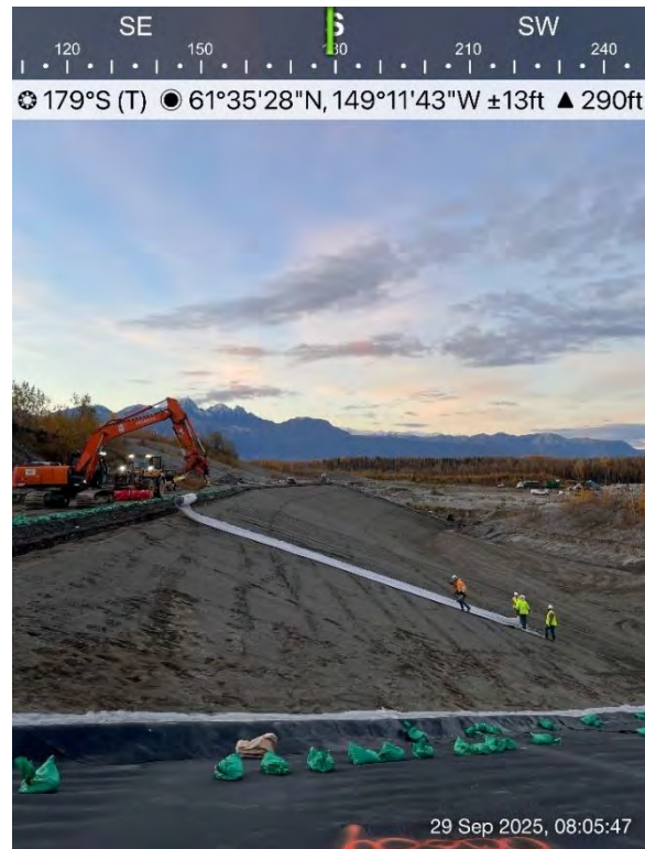
Figure 10: 09/29/25 - Cell 4 Expansion GCL Placement Day 2
