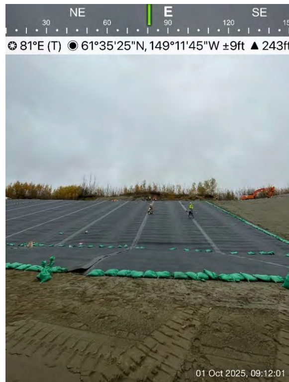
Figure 20: 10/01/25 - Cell 4 Expansion HPDE Geomembrane Liner Placement Day 4
