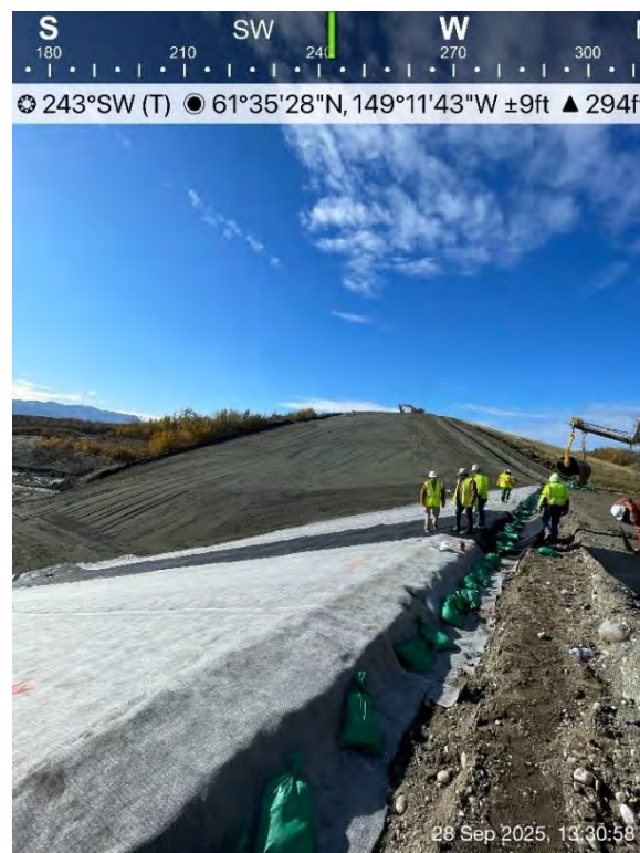
Figure 6: 09/28/25 - Placement of HDPE on the Northern Slope of Cell 4 Expansion with a Spreader Bar
