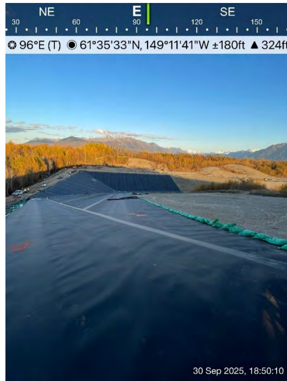
Figure 18: 10/01/25 - Cell 4 Expansion GCL Placement Day 4
