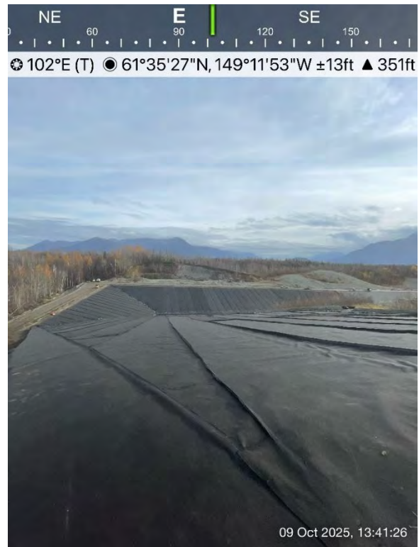
Figure 42:10/09/25 – Cell 4 Expansion Geotextile Cushion Placement Day 2
