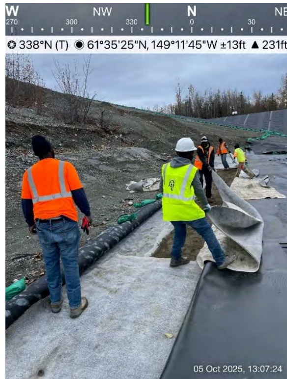
Figure 30: 10/05/25 – Cell 4 Expansion HDPE Liner Extrusion Welded to Existing Cell 2B HDPE Liner
