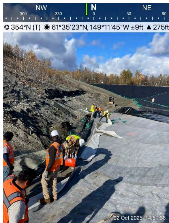
Figure 22: 10/02/25 - Cell 4 Expansion GCL Overlapped with Existing Cell 2B GCL
