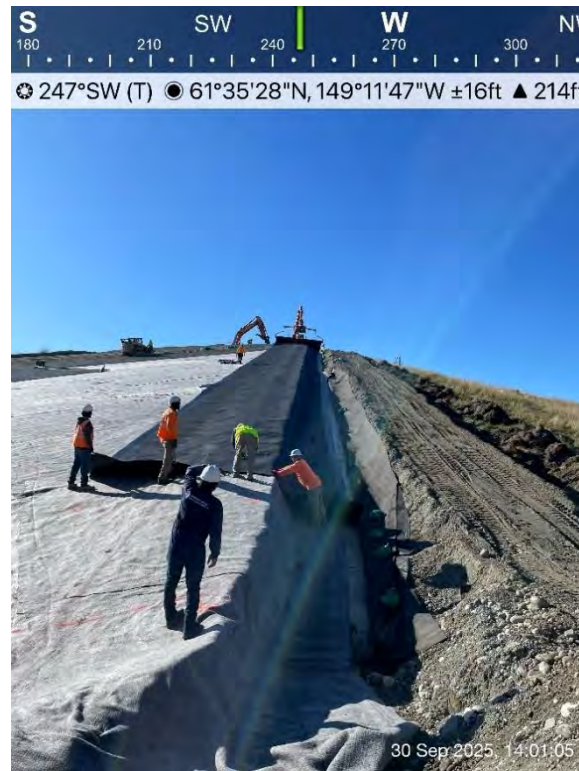
Figure 16: 09/30/25 - Cell 4 Expansion Extrusion Welding a Patch Over Air Test Holes
