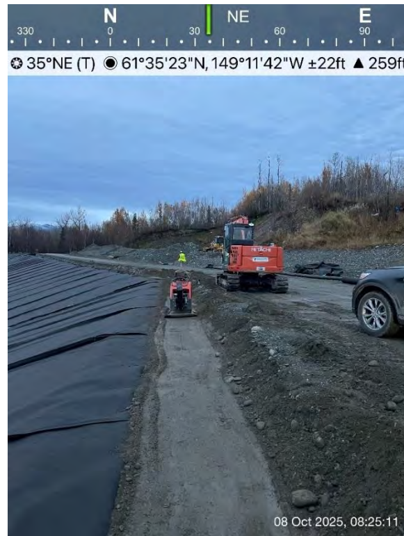
Figure 34: 10/07/25 - Cell 4 Expansion Geotextile Cushion Deployment with Spreader Bar
