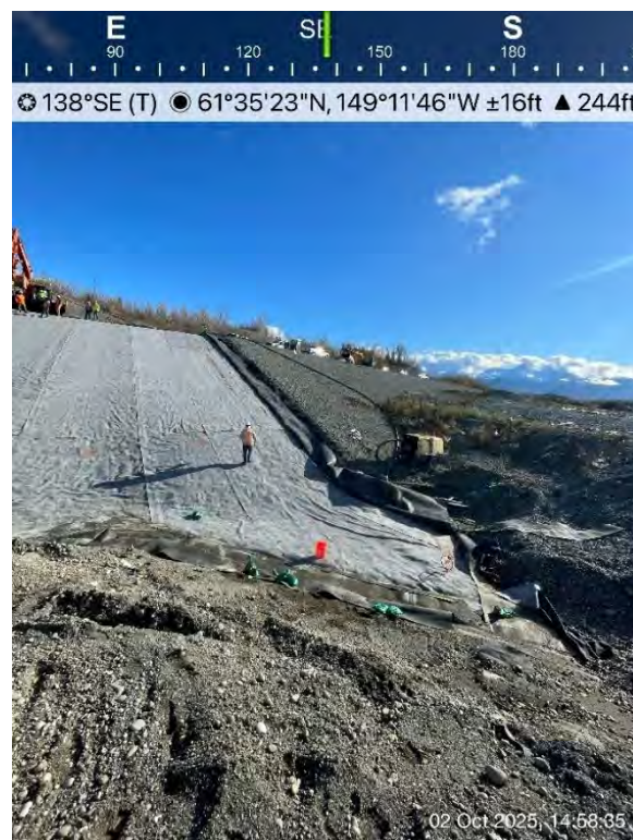
Figure 24: 10/02/25 - Cell 4 Expansion GCL Placement Day 5
