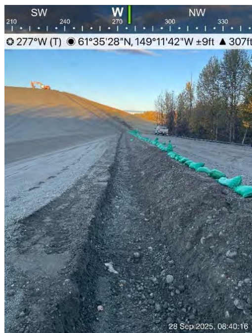
Figure 2: 09/28/25 - Cell 4 Expansion Termination Berm Trench
