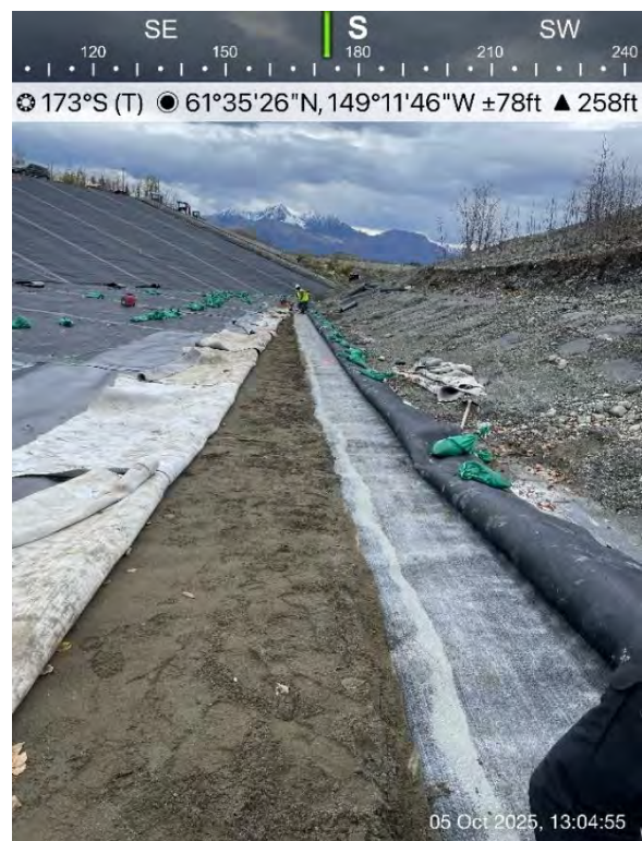
Figure 28: 10/05/25 – West Side of Existing Cell 2B GCL Exposed and Sprinkled with Granular Bentonite
