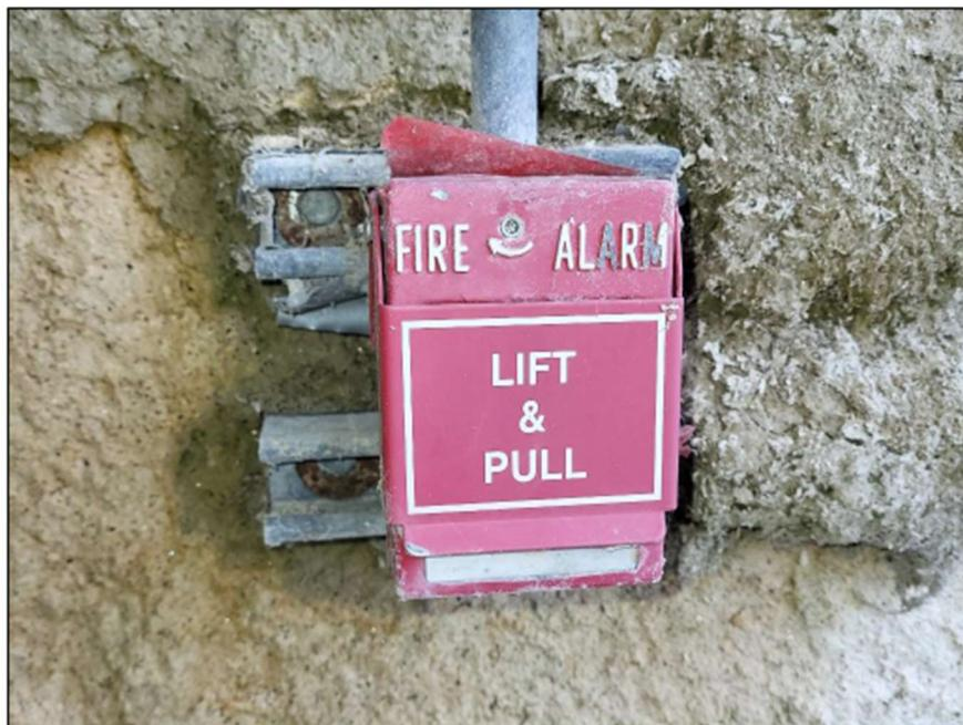
2. Sheet U3 Construction note B "UL-864 Listed Fire Alarm must be replaced In-Kind..." This appears to be a custom shop build FACP. Protect wire has a custom build option for a similar system. Existing protectowire is very likely conventional linear heat and would be compatible with any listed conventional FACP utilizing standard IDC inputs. Could bidders propose several conventional options compatible with existing protectowire.
