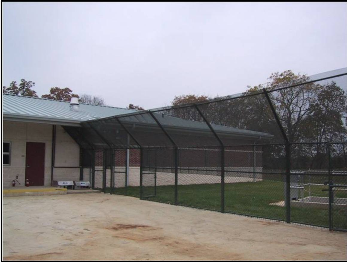
Figure 2-3: Welded Wire Mesh Fence
