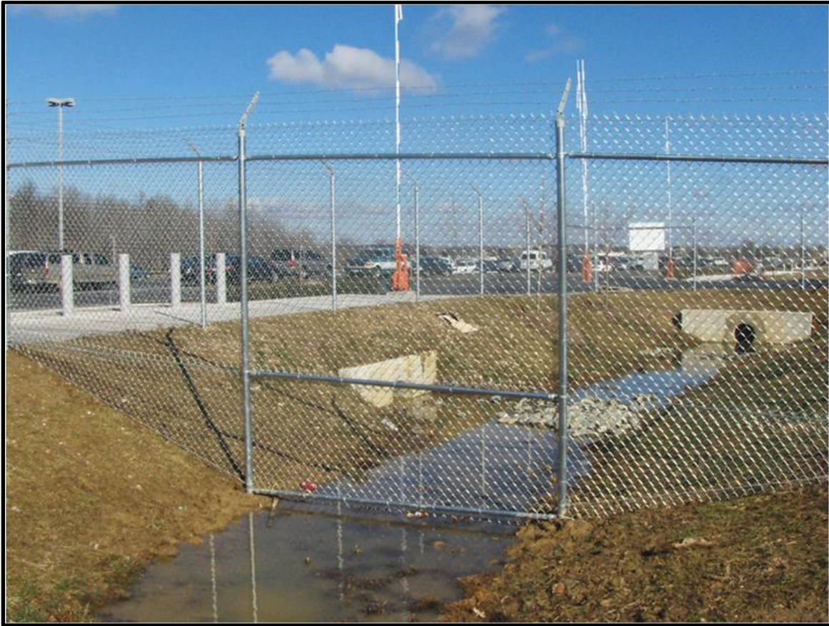
Figure 2-15- Chain Link Fence over Ditch
