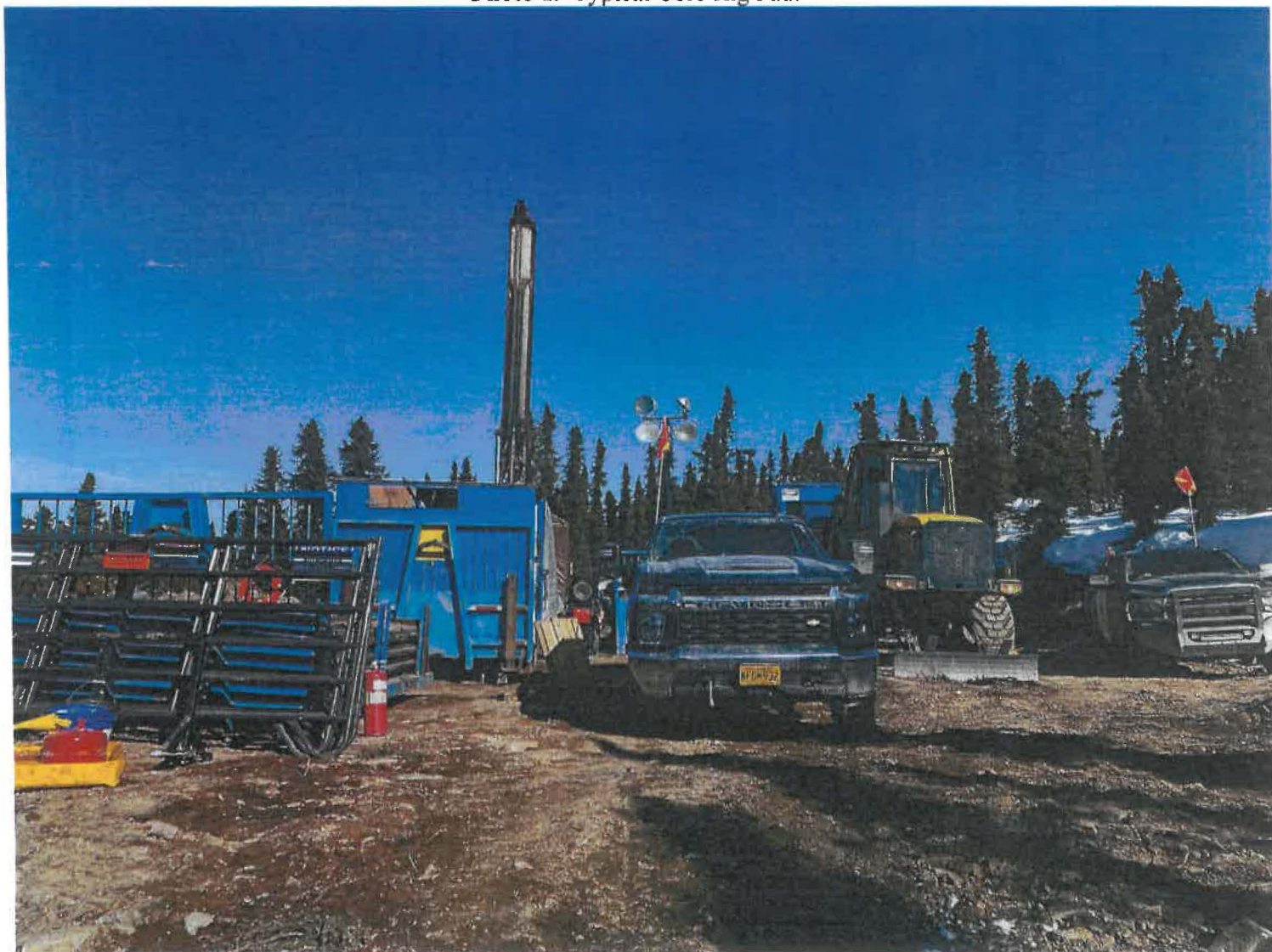
Photo 1. Typical Core Rig Pad.
