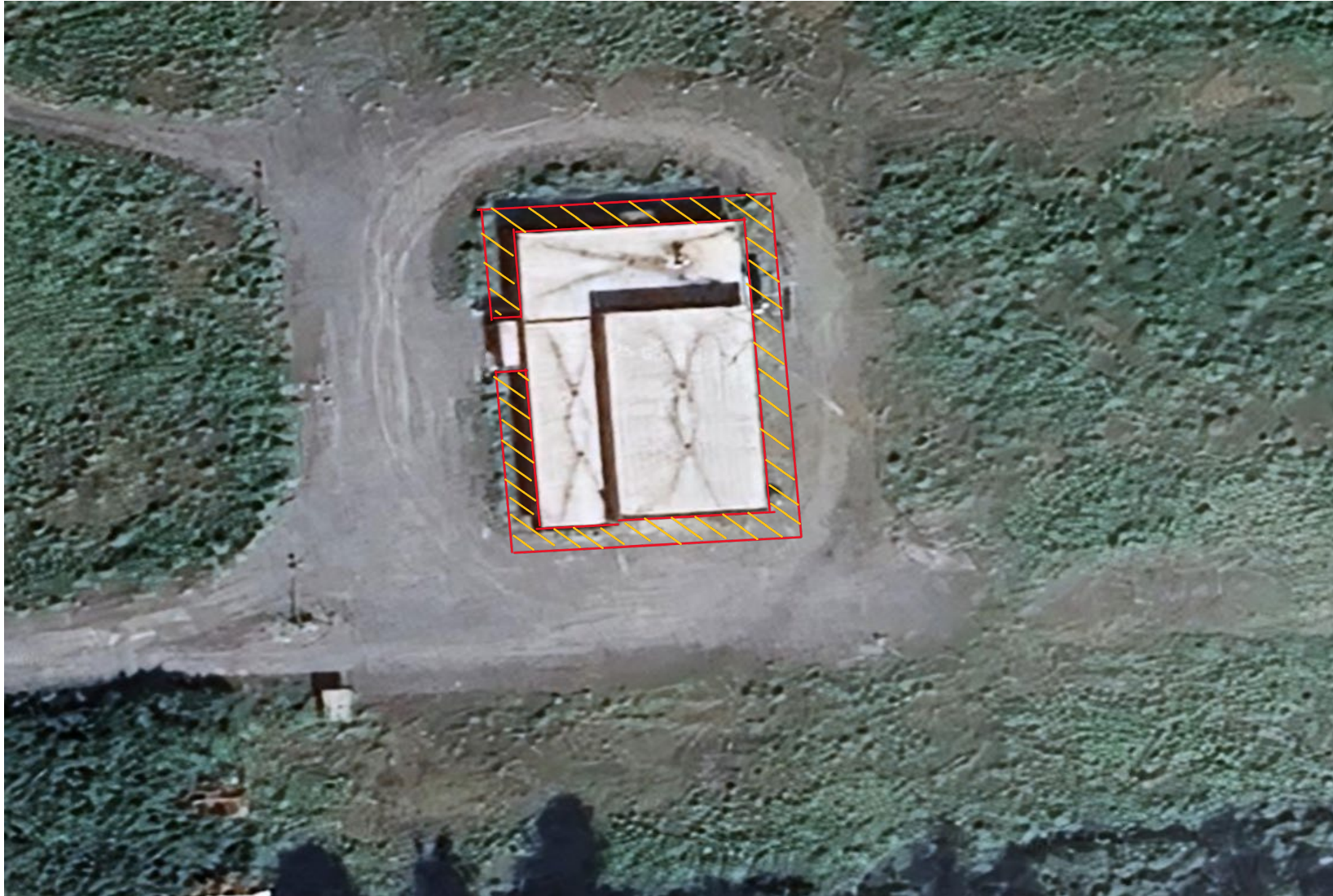
Attachment 13: Asphalt Apron around Building
