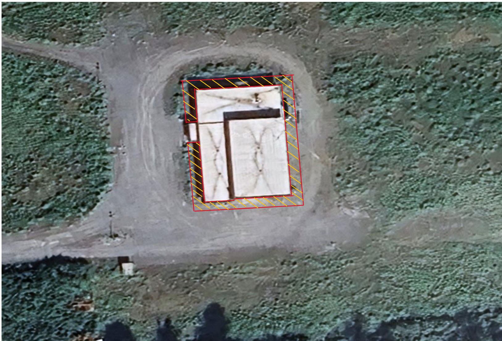
Attachment 13: Asphalt Apron around Building
