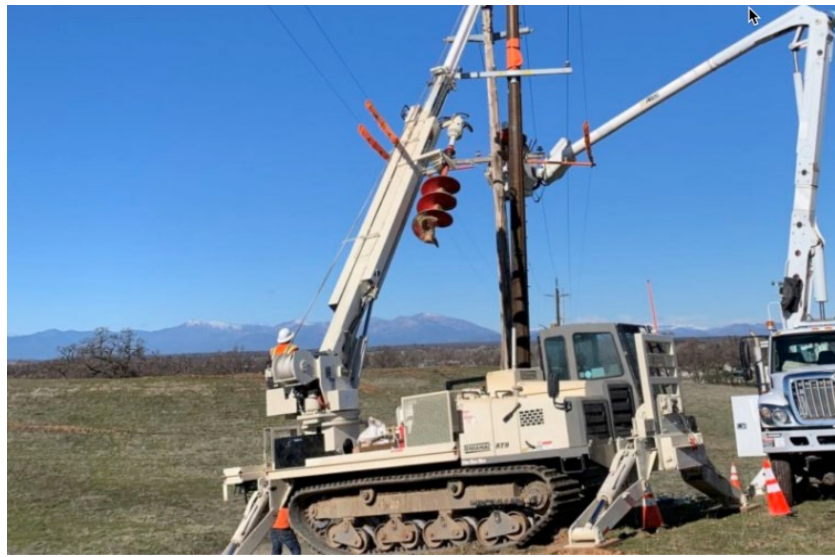
Figure 27: Aerial Pole Construction
