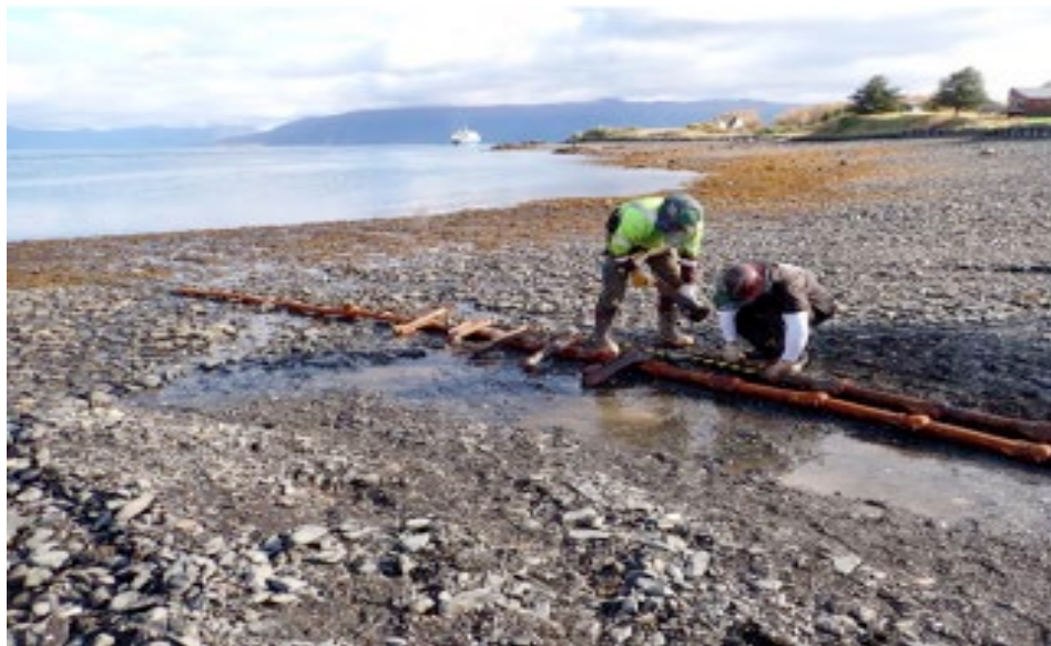
Figure 11: Articulated Pipe being installed
