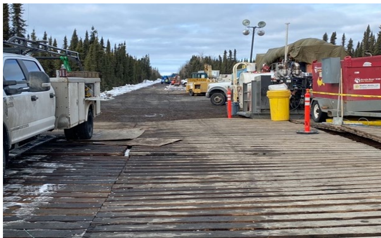
Figure 19: Drill mat “road”
