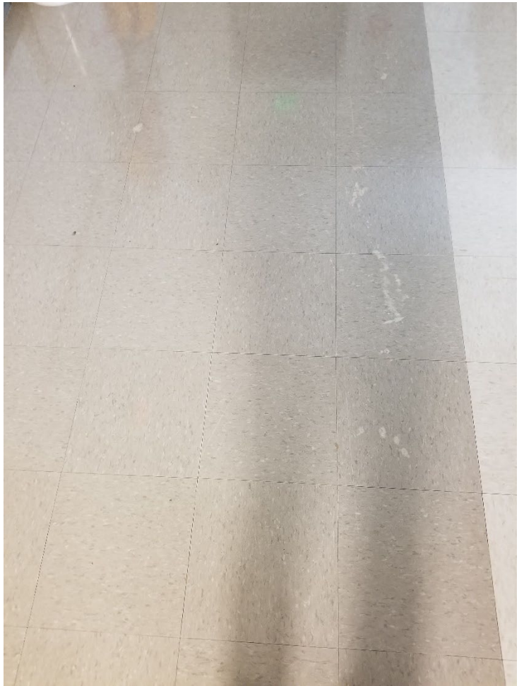
Hallway/Large Office Flooring
