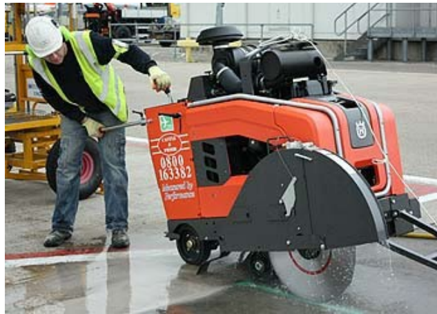
Figure 14-3 Diamond Blade Sawing
