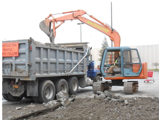
Figure 14-5 Concrete Removal Using Backhoe
