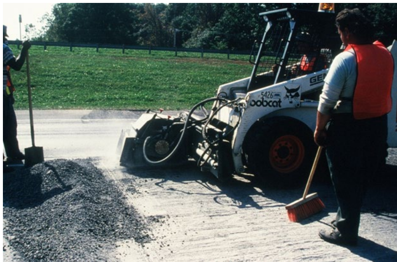
Figure 3-4 Small Milling Head Attachment
