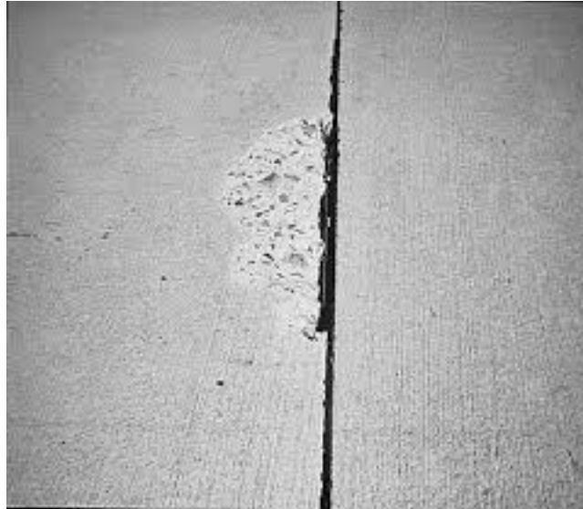
Figure 13-2 Incompressible Causing Spalling at a Joint or Crack
