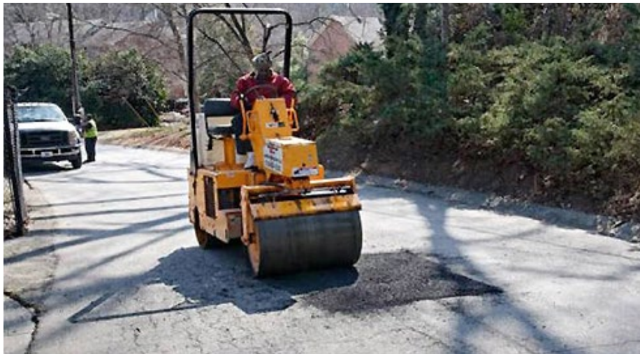
Figure 3-9 Check Level of Patch Surface
