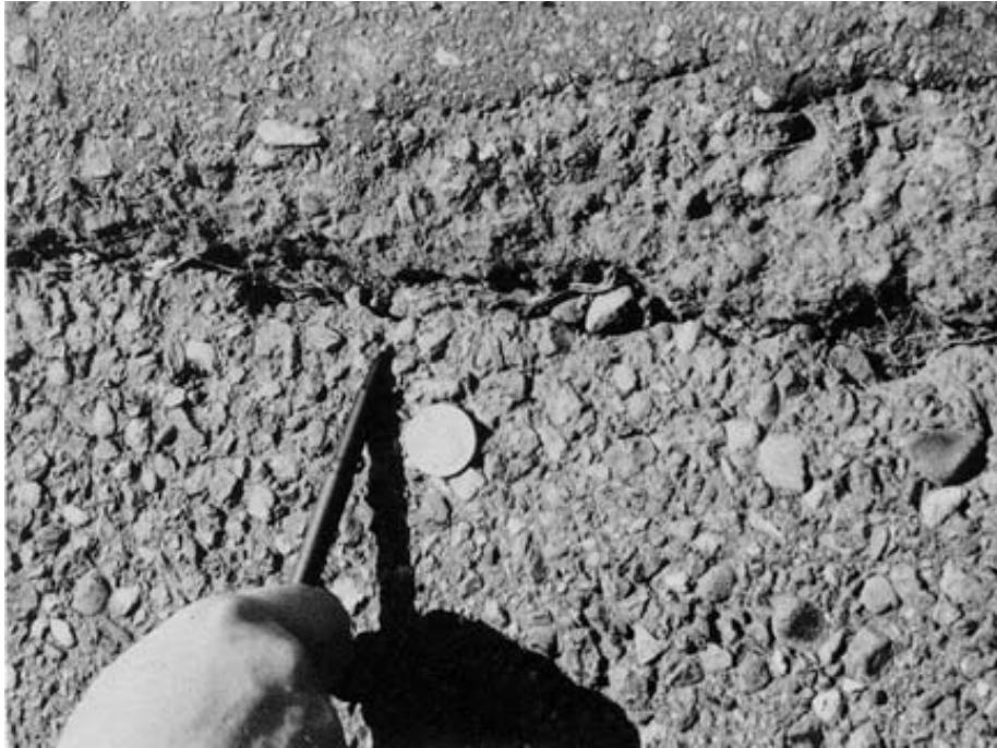
Figure 9-7 Large Crack
