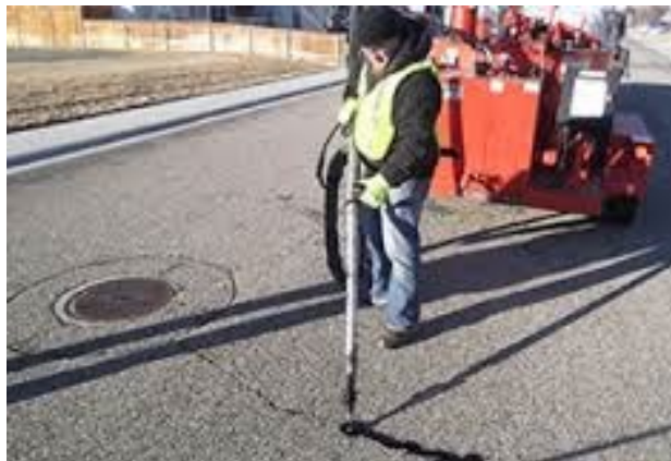
Figure 9-9 Filling Crack with Sand Emulsion Mixture
