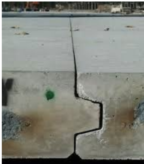
Figure 18-8 Keyed Joint
