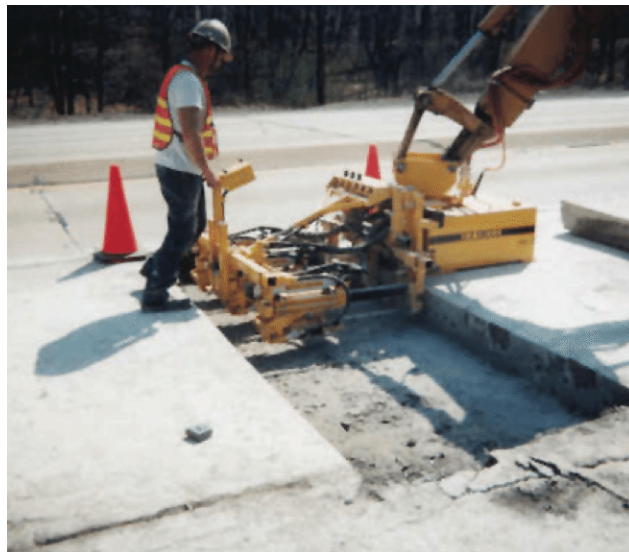
Figure 18-9 Gang-operated Dowel Drill
