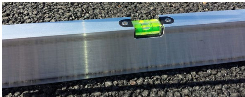
Figure 3-9 Check Level of Patch Surface
