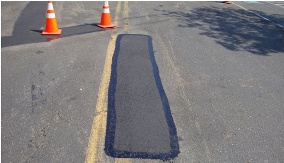
Figure 3-10 Seal the Edges
