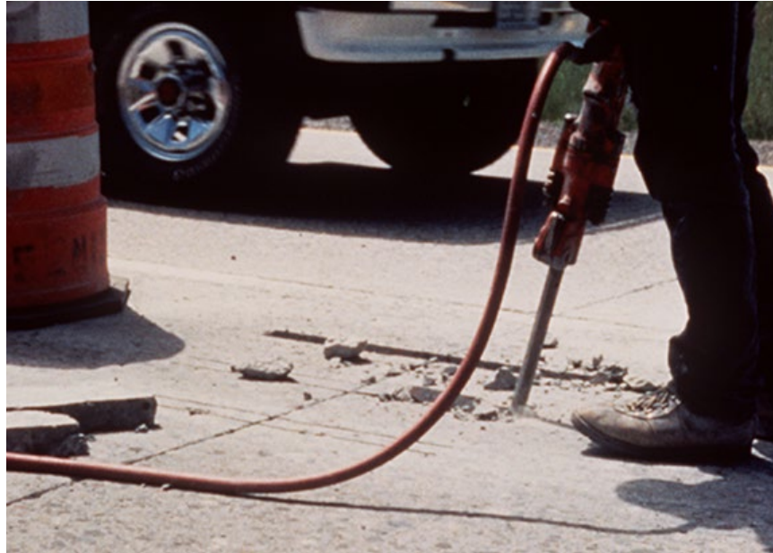
Figure 18-5 Use of Chipping Hammers to Remove Concrete
