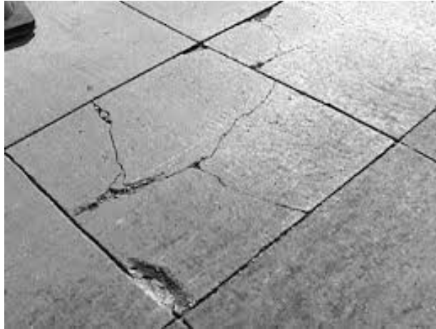
Figure 14-1 Shattered Slabs
