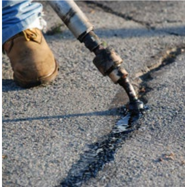
Figure 9-11 Sealing the Crack
