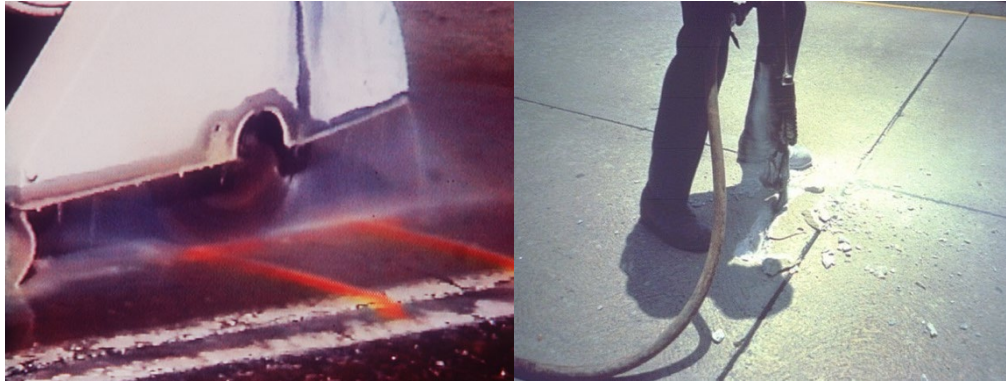
Figure 13-5 Repair Boundary Sawing and Use of Chipping Hammer
