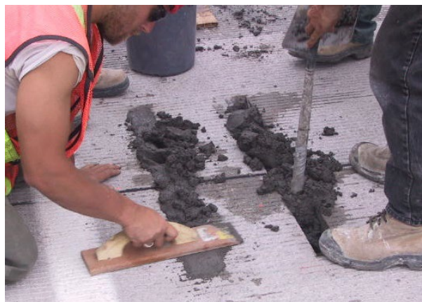
Figure 18-7 Placing and Consolidating Patch Material
