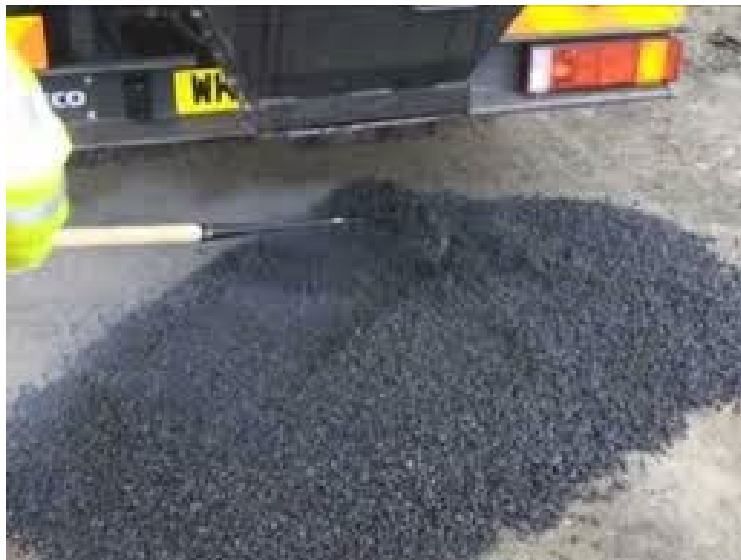
Figure 3-6 Overfill Prior to Compaction
