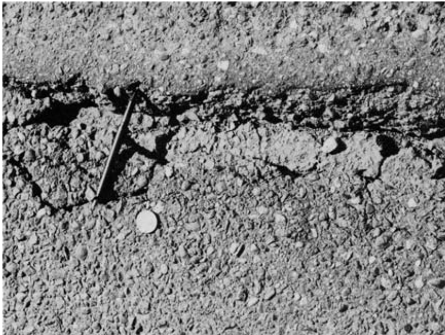
Figure 9-7 Large Crack
