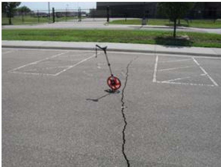
Figure 9-3 Longitudinal Cracking
