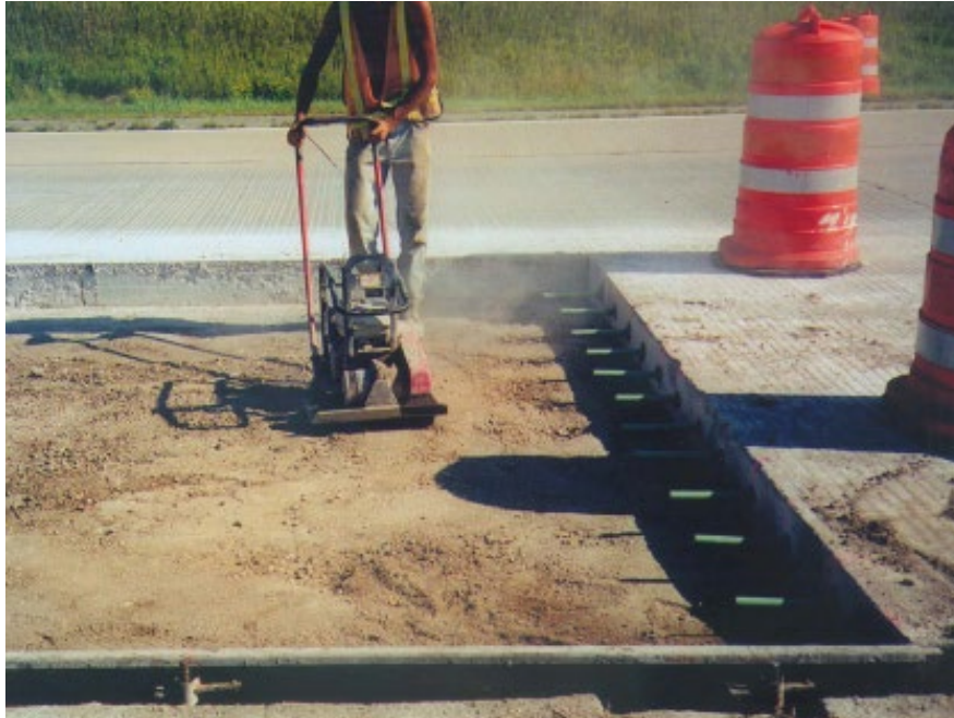
Figure 14-9 Patch Area Compaction
