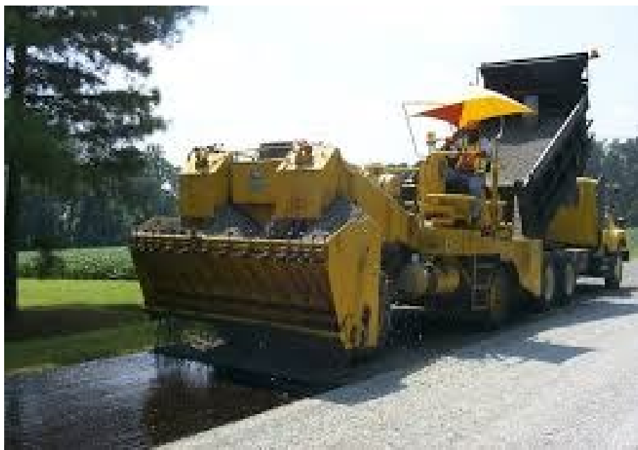
Figure 6-2 Applying Aggregate with Self-Propelled Hopper-type Spreader
