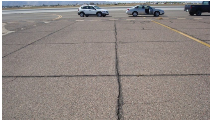
Figure 9-3 Longitudinal Cracking
