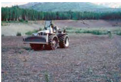
Figure 102: A landfill compactor being used to loosen and imprint the surface of an old gravel pit.
