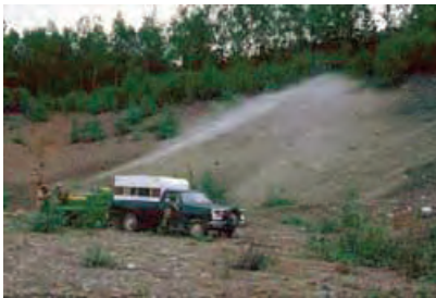
Figure 87: A small tow-behind hydroseeder in use.
