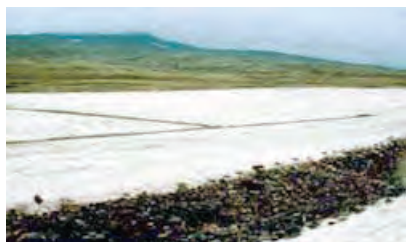
Figure 89: Well-placed excelsior blankets being used to control erosion prior to vegetation growth.
