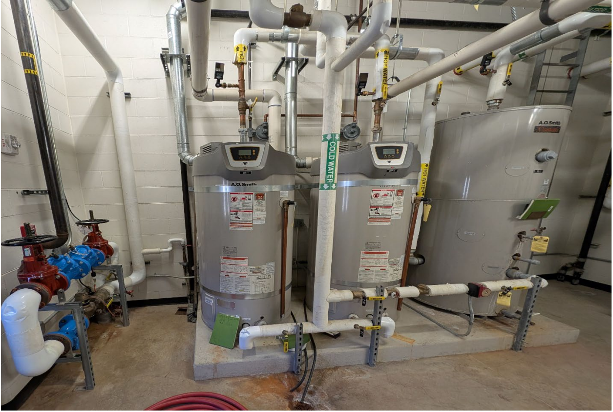
Figure 4: East facing view of mechanical room
