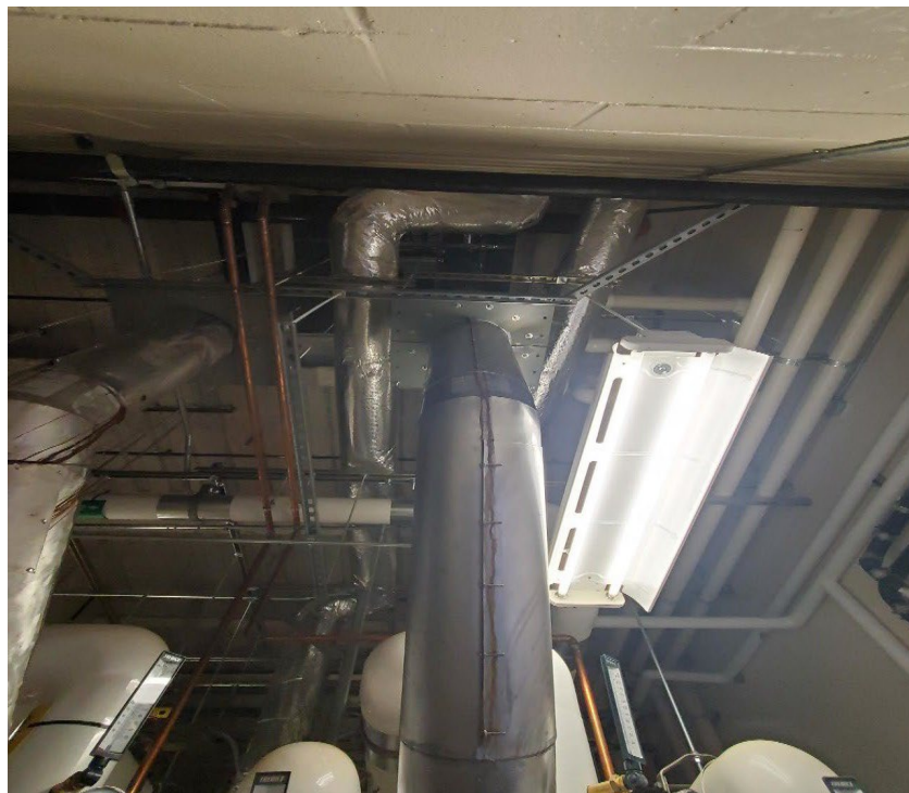
Figure 4. Routing of vent to roof
