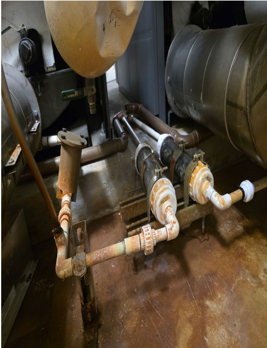
Figure 5. Condensate drain assemblies
