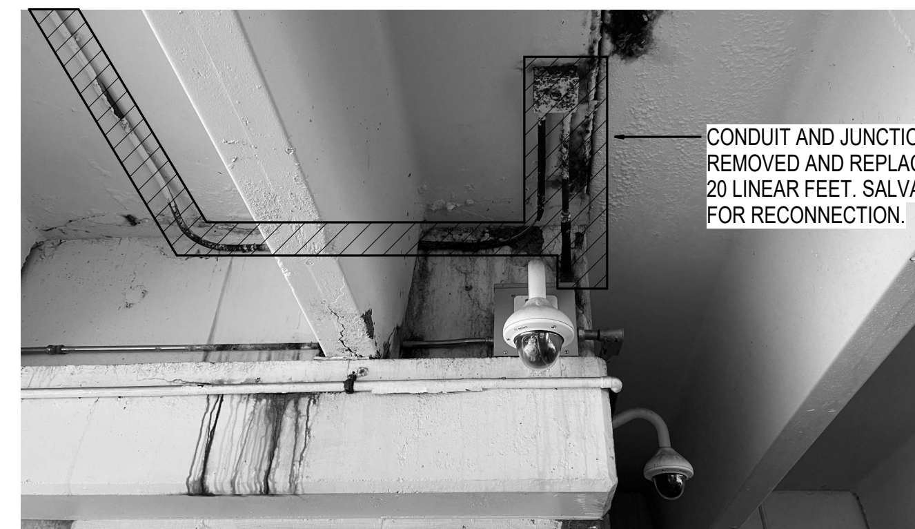
3 CORRODED CONDUIT PHOTO NOT TO SCALE
