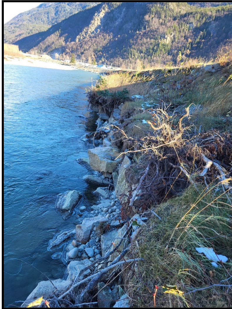
Figure 6 – Erosion along toe where airport modification was complete in 2001. Area should have a 13-foot-wide toe and the toe is only roughly 3 feet wide in this section.
