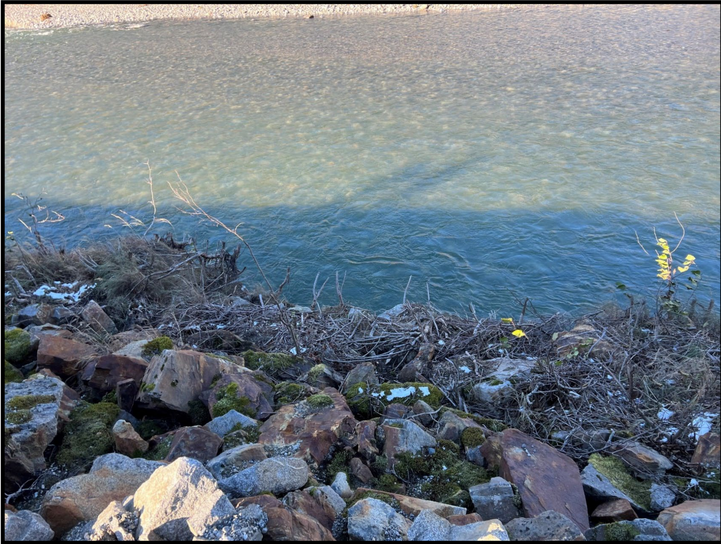
Figure 8 – One of the areas along the levee where the toe is completely gone from erosion. Scour and undermining of the structure is beginning to occur.
