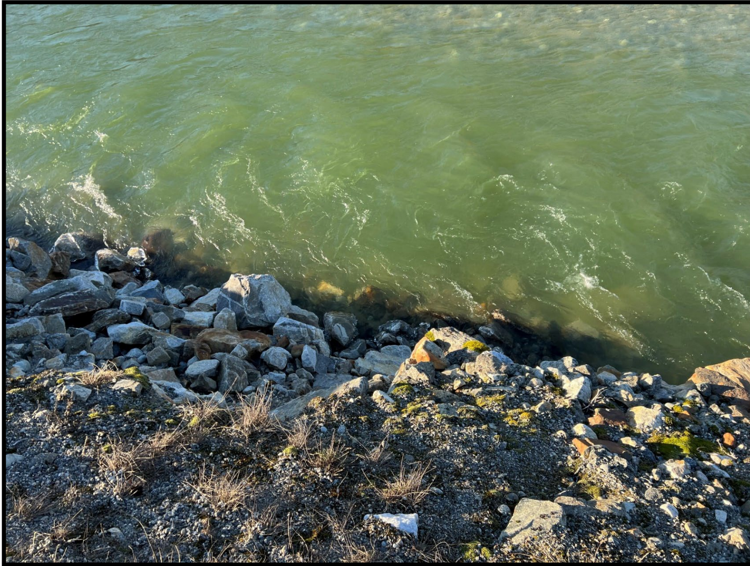
Figure 9 – Toe has been completely eroded along this stretch of the levee with slopes near vertical. Embankment is starting to slide.
