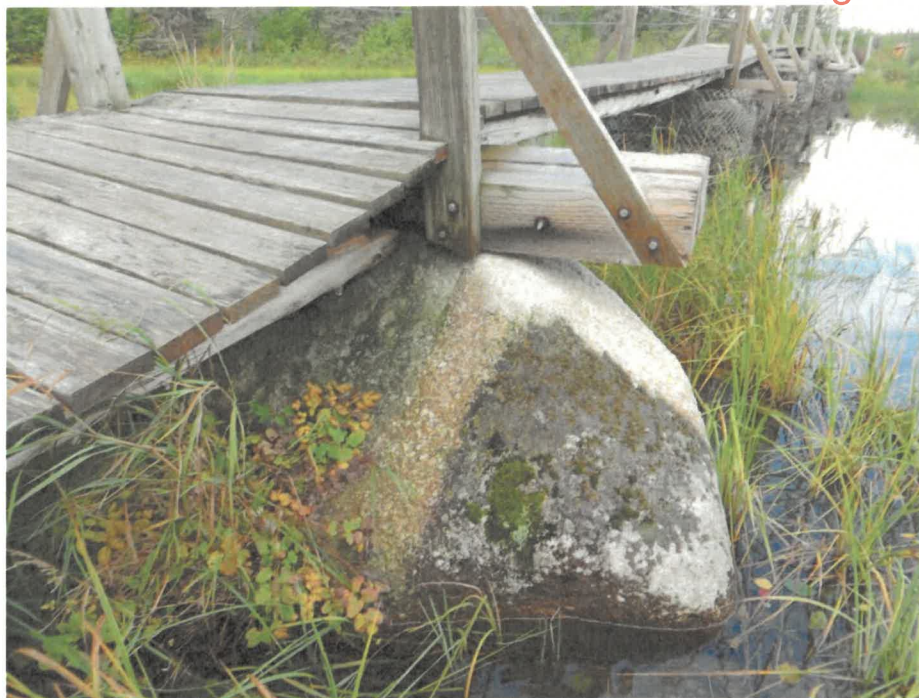
Figure 5. Boulder Foundation (September 7, 2017)
