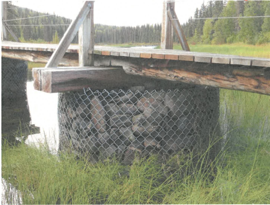
Figure 3. Rock Foundation (September 7, 2017)
