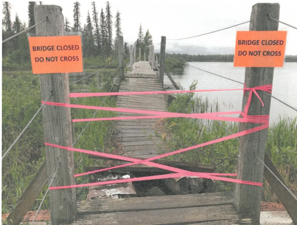
Figure 8. Bridge Closure (June 20, 2020)
