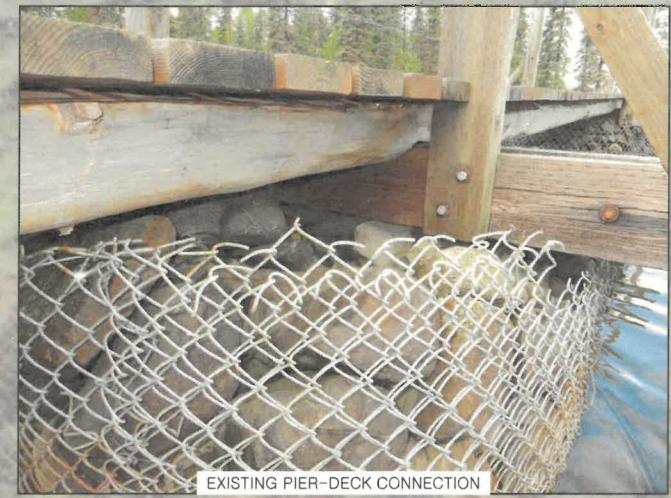
EXISTING PIER-DECK CONNECTION
