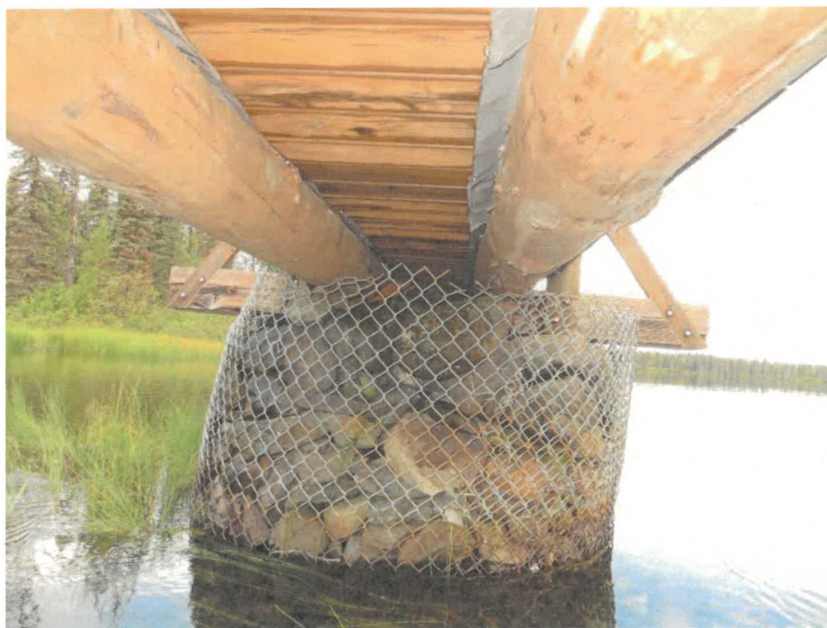
Figure 6. Bridge Underside (September 7, 2017)
