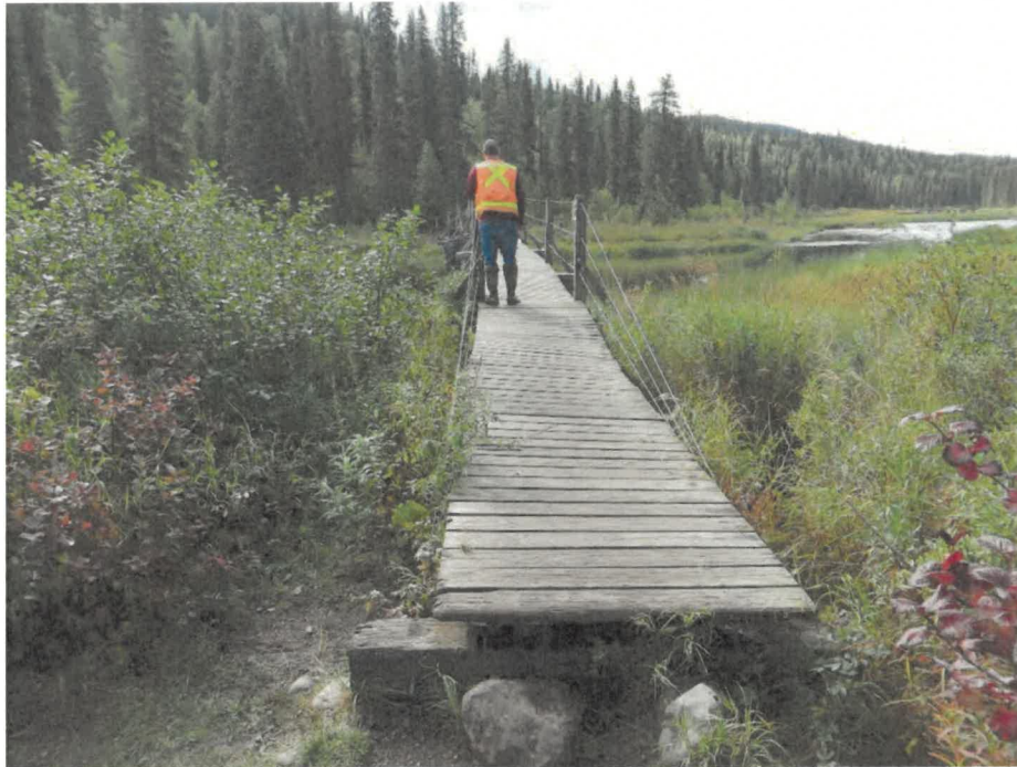
Figure 1. Bridge Conditions Facing South (September 7, 2017)
