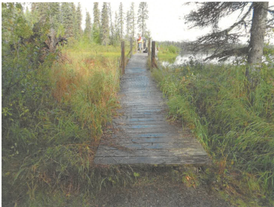
Figure 2. Bridge Conditions Facing North (September 7, 2017)
