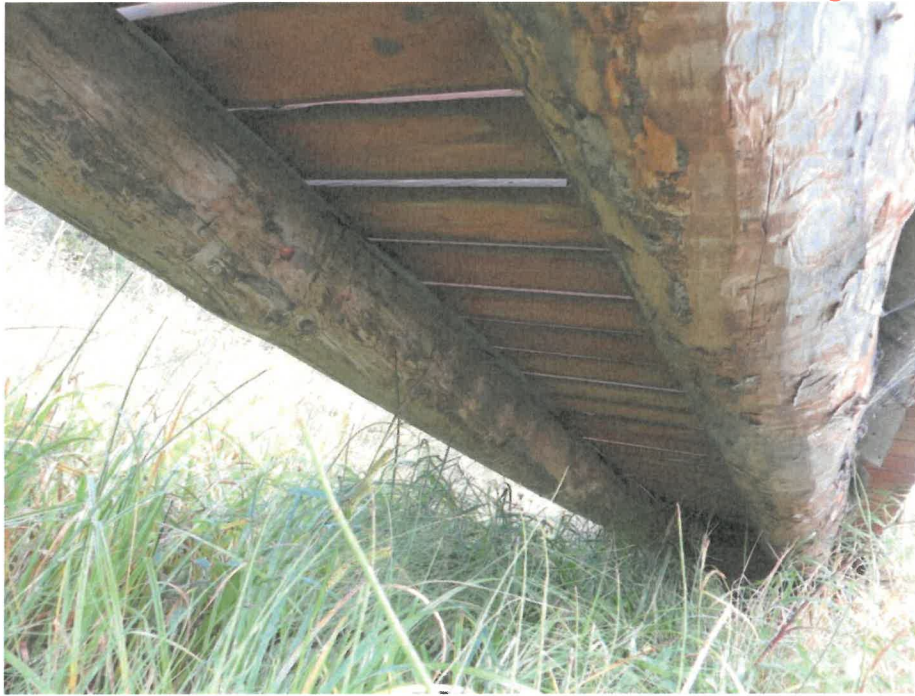
Figure 7. Bridge Ramp Underside (September 7, 2017)
