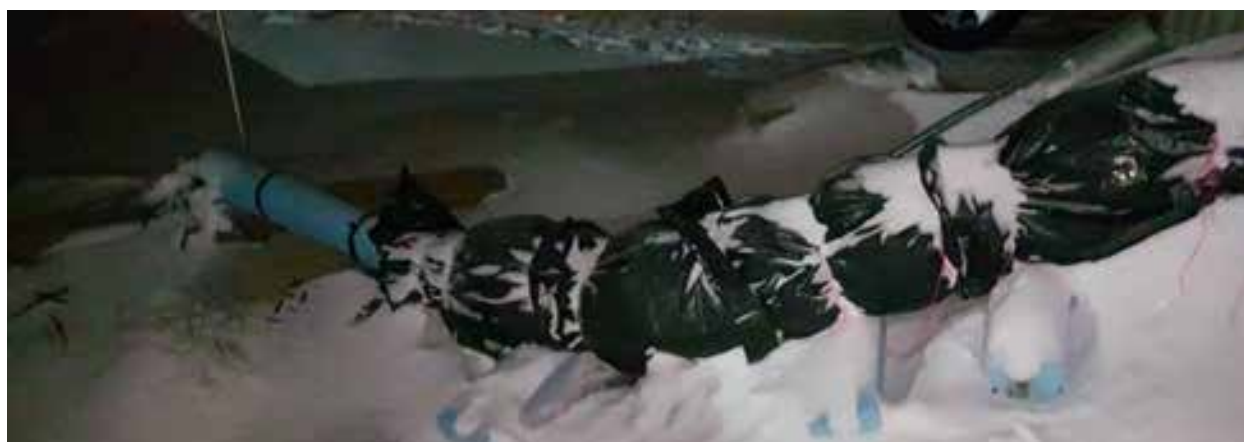
Figure 12 - Another view of the temporary lift station bypass
