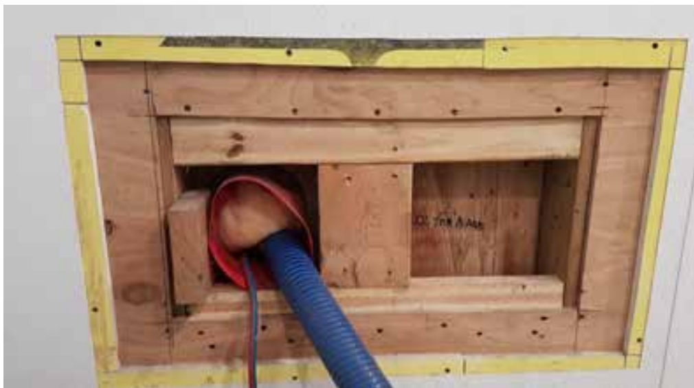
Figure 9 - Interior View of Temporary Lift Station Bypass
