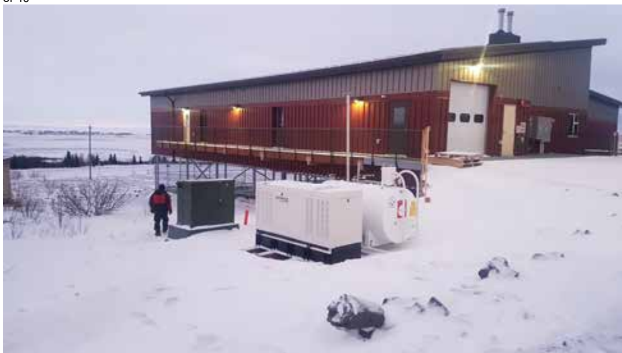
Figure 47 - Elders Home under Construction
