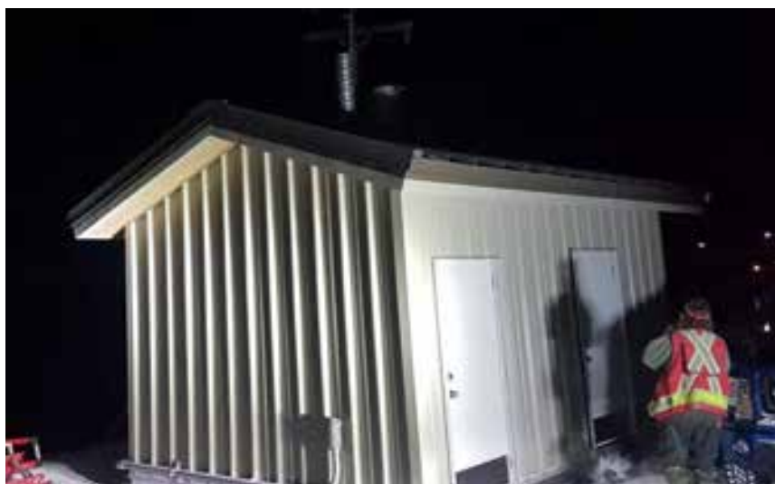
Figure 10 - Exterior View of HVLS
