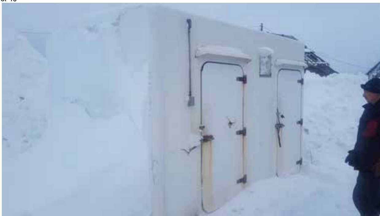
Figure 35 - Covenant Lift Station exterior
