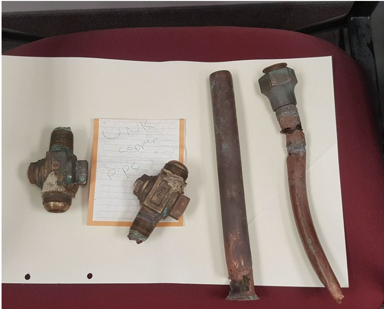
Figure 2.2: Pitorifices and Piping Typical Failures
