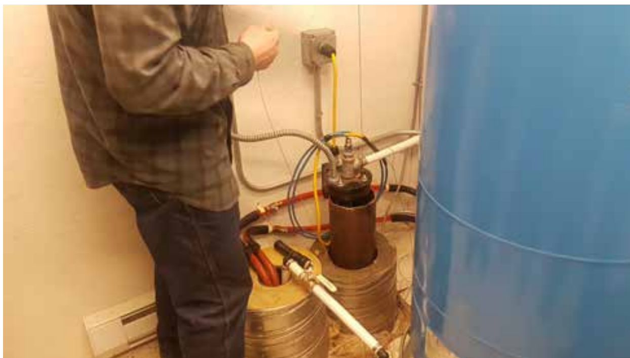
Figure 48 - Elders Home Pump House - attempting to set new data logger after existing one fell down during removal
