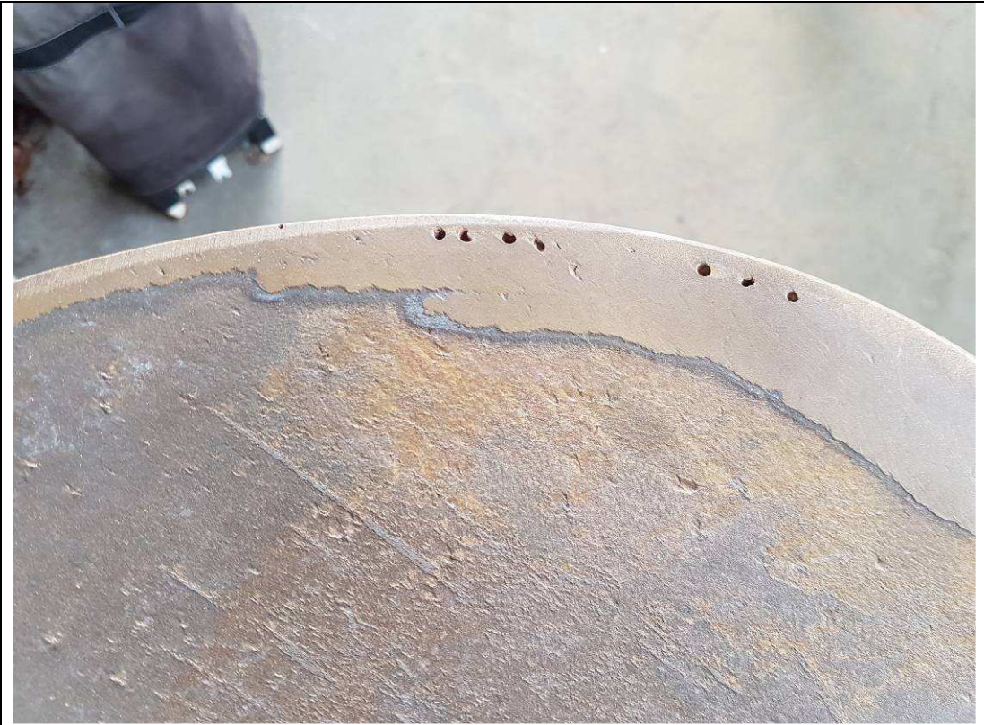
Photo of previous weld repair, with pin holes.
