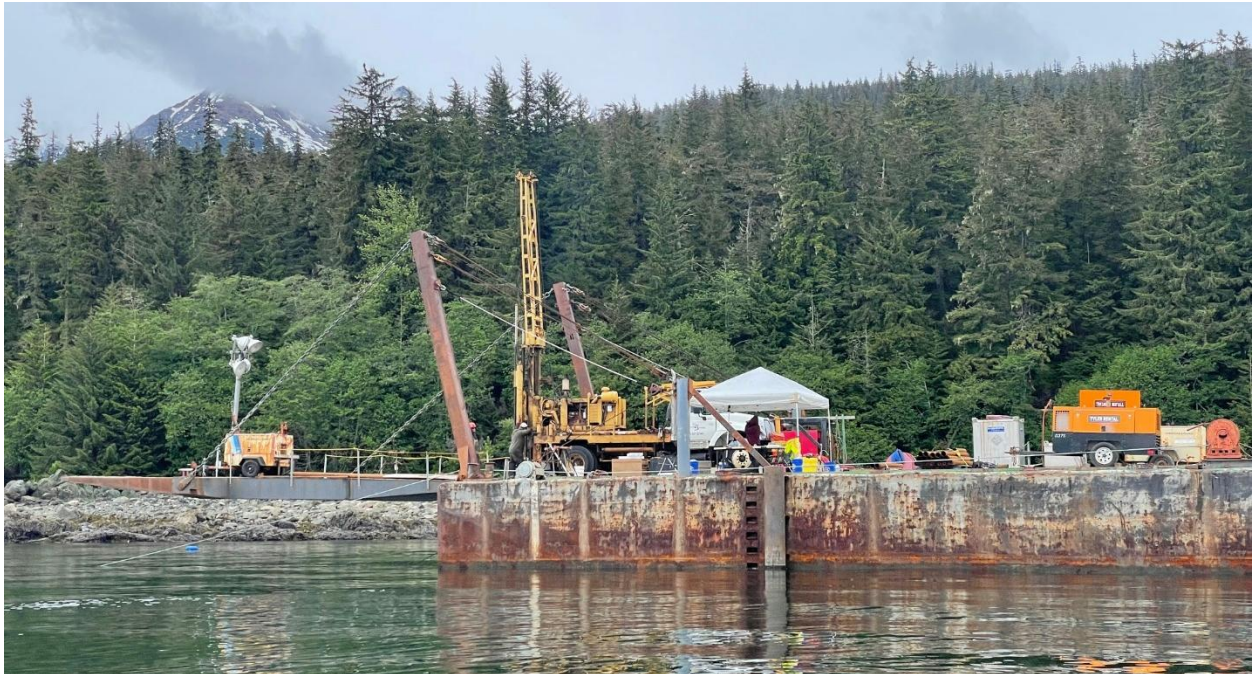
Figure 5. Closeup of the Drill Mounted on a Truck on a Ramp Barge
