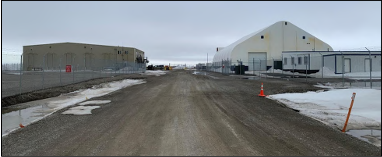
Figure 4-8: Road to Wright Air Terminal/Hangar where Snow Removal is Problematic
