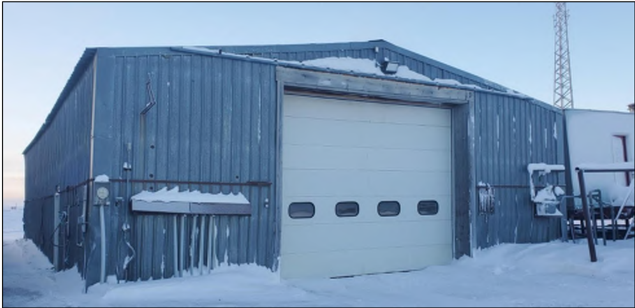
Figure 4-5: Aged M&O Cold Storage Building
