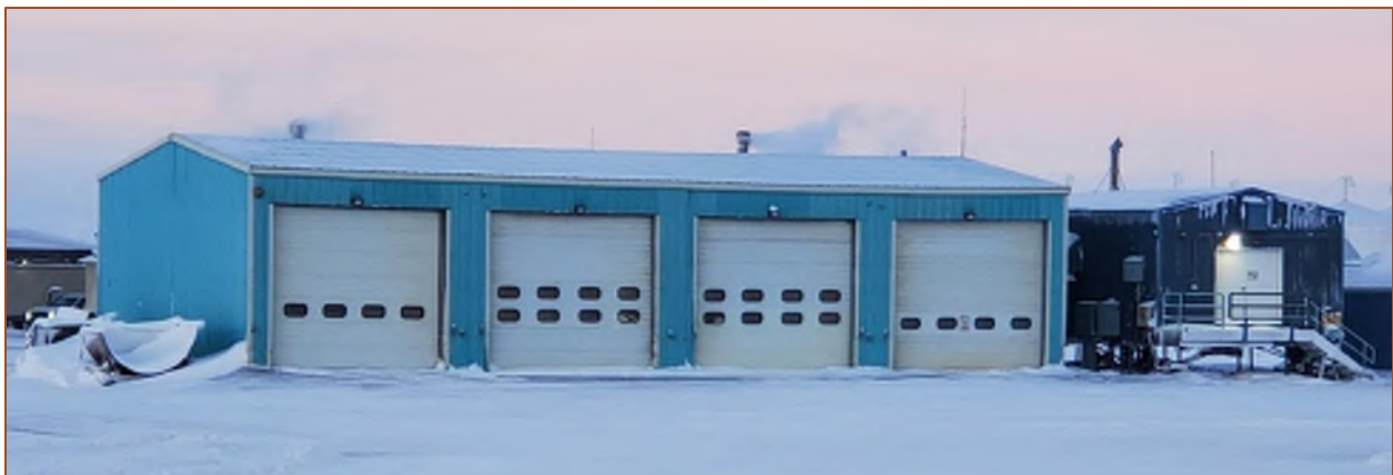
Figure 4-6: Aged M&O Warm Storage Building
