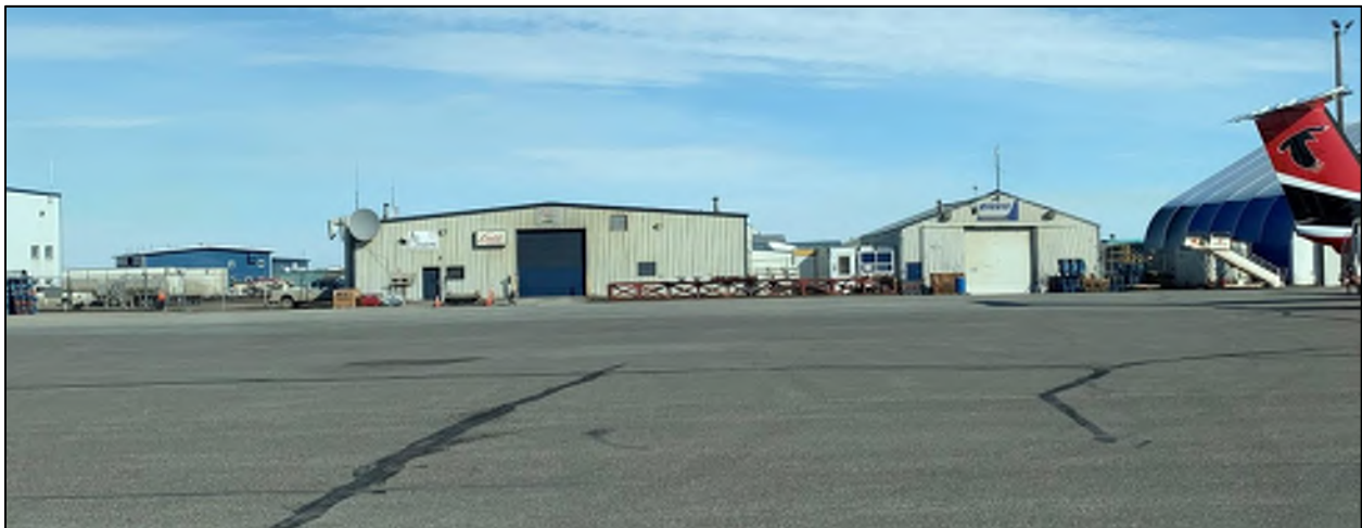
Figure 2-8: Carlile Lease Lots From Airside, on Terminal Apron
