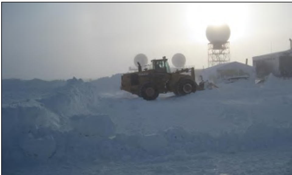
Figure 2-15: Snow Buildup between buildings at SCC
