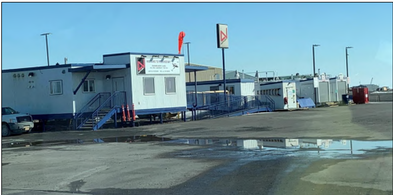
Figure 2-14: Colville Fueling Apron
