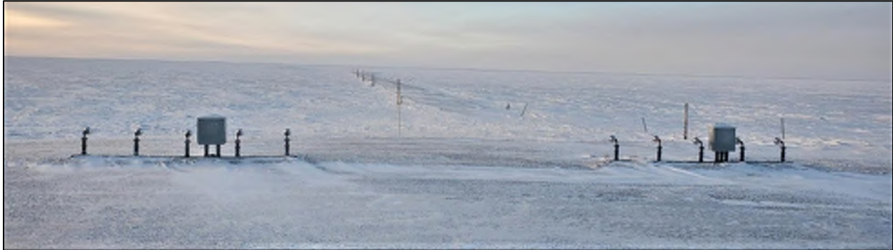
Figure 2-4: Runway 6 Threshold and Approach Lights
