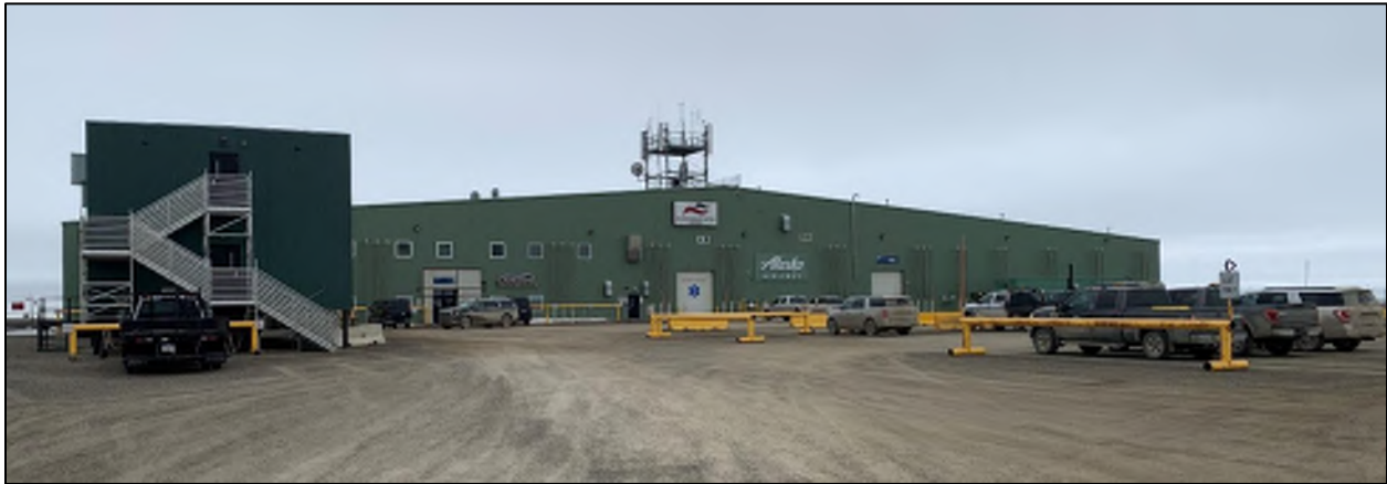
Figure 2-11: Deadhorse Aviation Center From Landside
