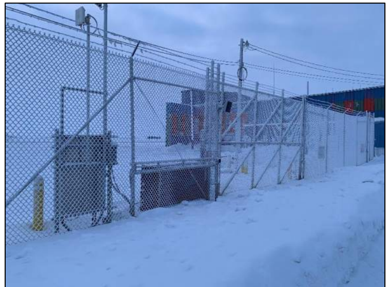
Figure 2-7. Security Fencing at BRW
