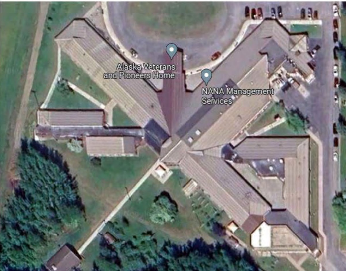
REFERENCE AERIAL PHOTOGRAPH
