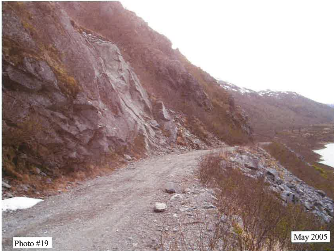
MP 2.4 - Rock fall from steep joints and exfoliation planes.
