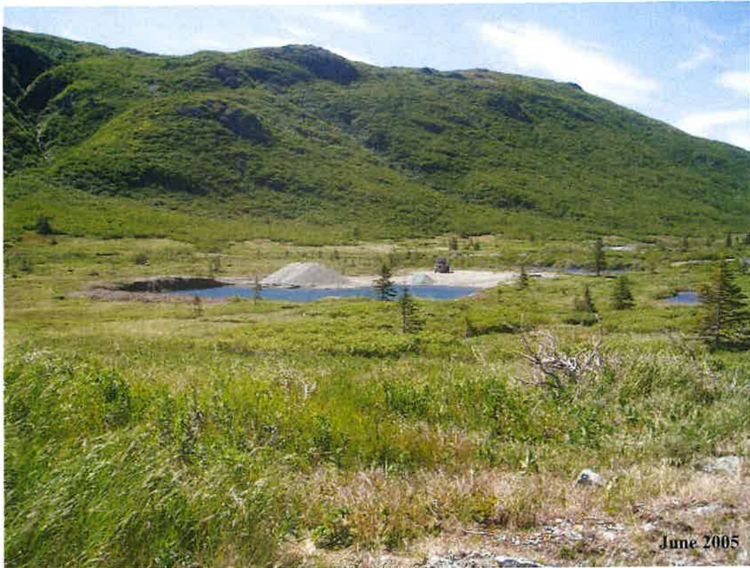
MP 3.9 - Looking at the existing material site at MP 4.0 from the road.
