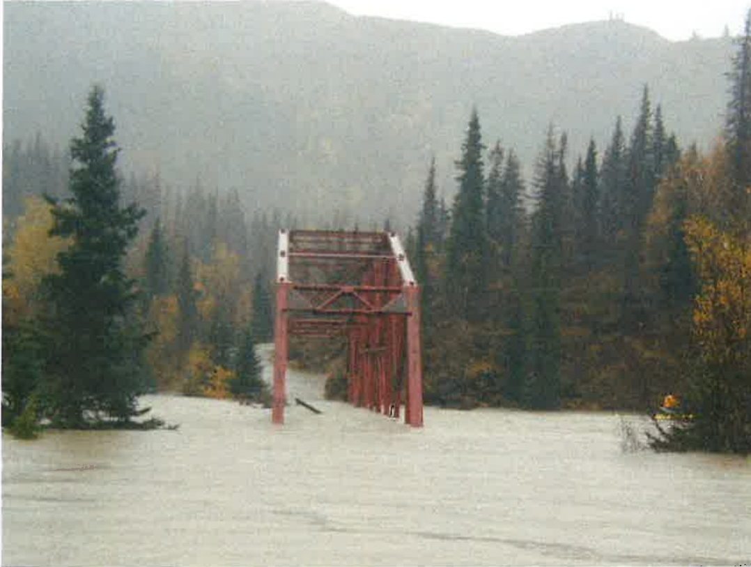
MP 11 - "old" bridge that crosses the Iliamna River at flood stage.
