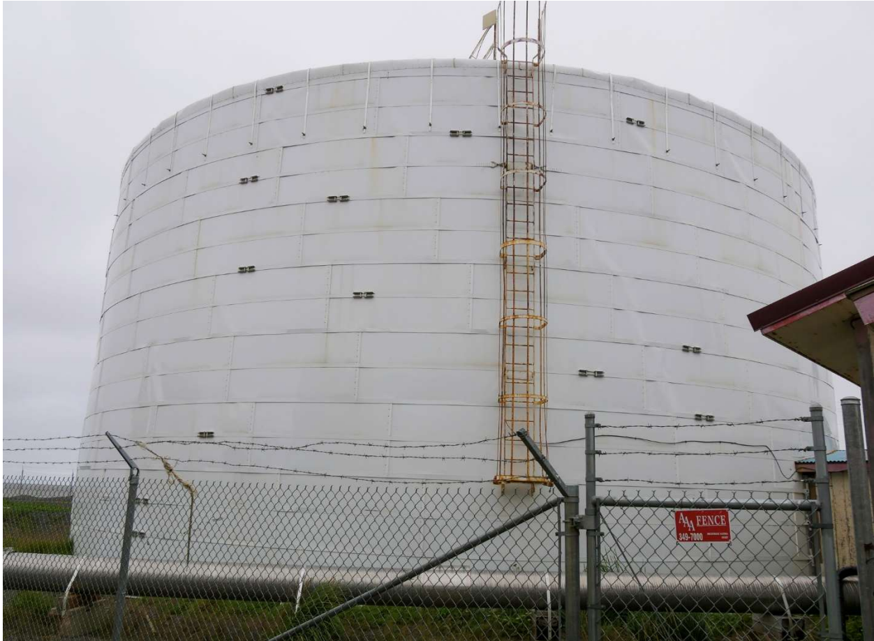
Figure 39: Shaktoolik community Water Storage Tank. A rehabilitation of the water storage tank was completed in the summer of 2015 which consisted of roof repairs, new exterior siding, and new insulation.
