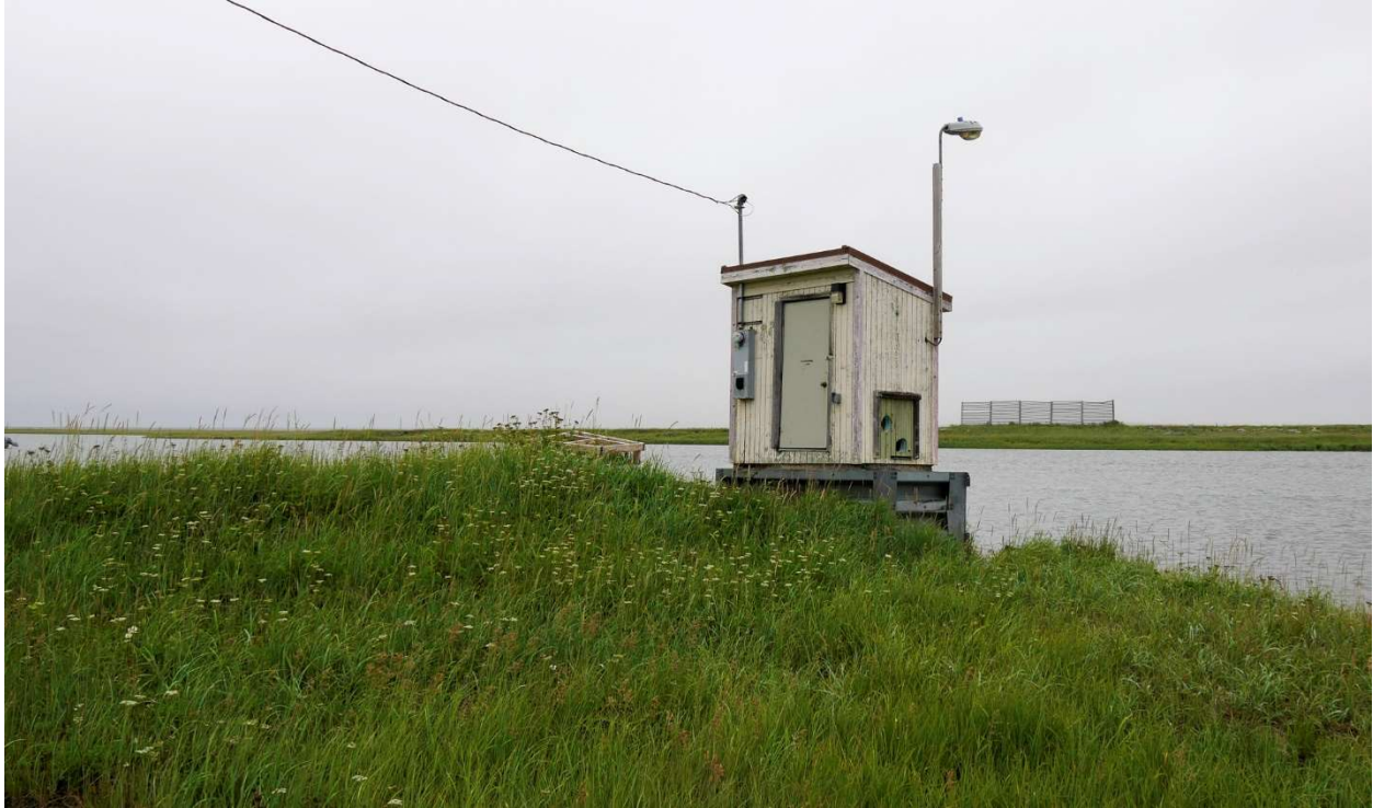
Figure 7: Winter water source pump house located adjacent to town along the Tagoomenik River.
