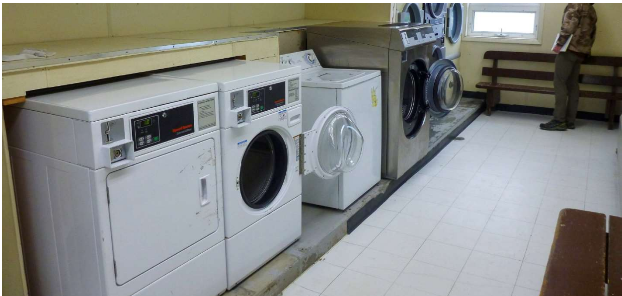
Figure 38: Inspection of washeteria (located within WTP).
