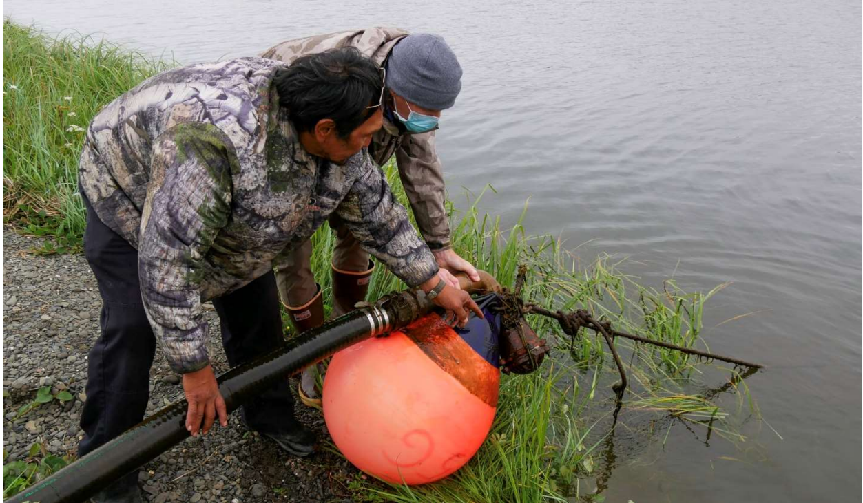
Figure 40: Water intake hose at the summer water supply approximately 6,500 feet south of the WTP. The summer supply provides water upstream of fish cleaning areas adjacent to the community, as well as upstream of the the community dump. The summer source is used as long as possible, with operators targeting ground freeze-up before switching to the winter water source.
