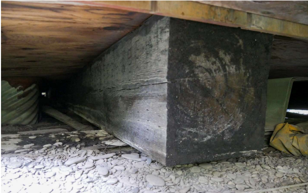
Figure 37: Photograph underneath the WTP. Timber beams lie on wooden footers on a gravel pad on grade to support the building and appear to be original construction.
