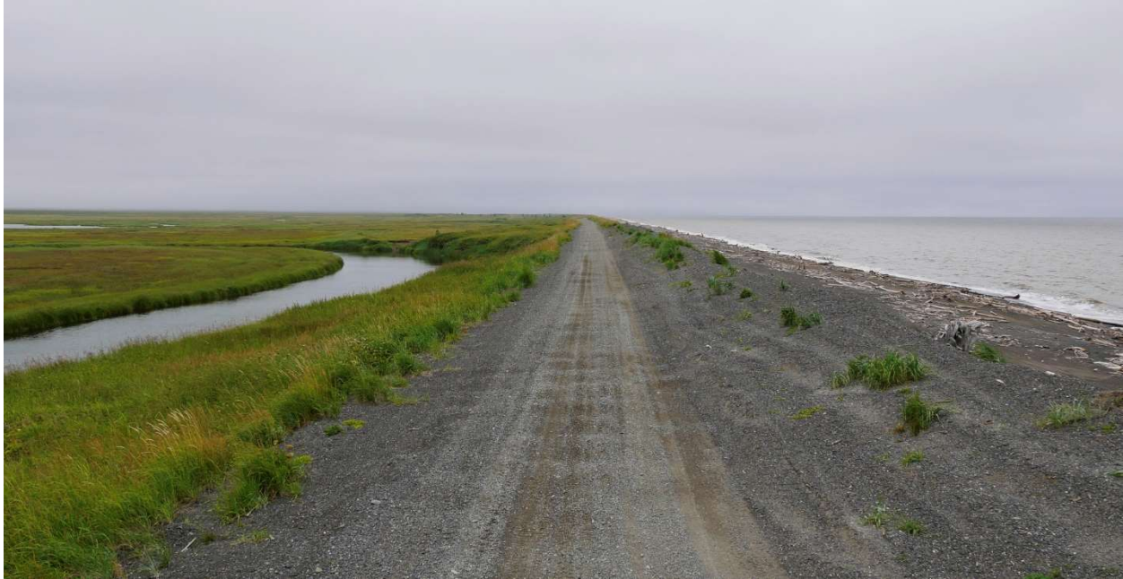
Figure 43: The most pressing threat to the community is “the berm” a narrow point approximately three miles south of town where an oxbow bend in the Tagoomenik river cuts dangerously close to Norton Sound. Storm surge flooding and waves from a large fall storm could possibly breach the berm and relocate the mouth of the river to this location, cutting Shaktoolik off from its summer and winter water supply points as well as a primary evacuation route. A permanent breach of the berm would likely require relocation of the community. A separate project is currently underway to study and reinforce the berm in this location.
