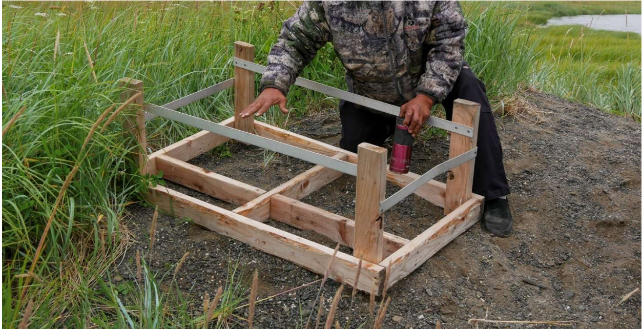
Figure 5: Winter water intake frame. In the winter, a hole is prepared in the ice and then covered with this wooden frame, which is packed in insulation to prevent the hole from refreezing. The foot valve is placed in the water, protected by the insulated wooden frame. The 100 foot long hose comes out of the insulated wooden frame and is routed to the pump house. An electric hair dryer is placed inside the insulated wooden frame to further protect from refreezing.
