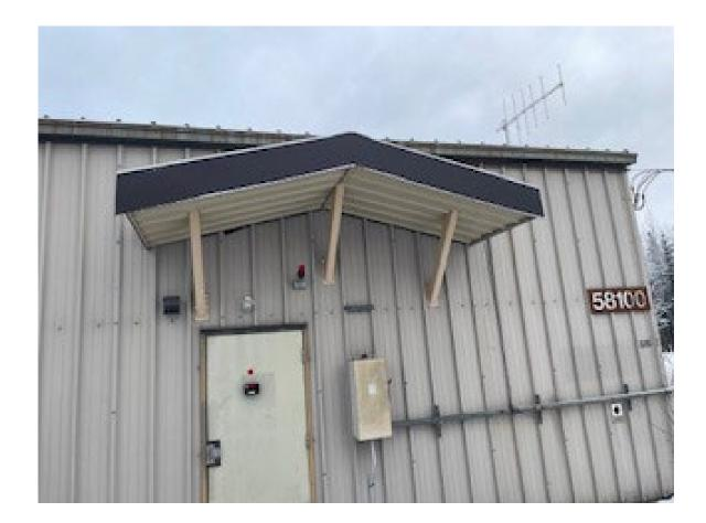
Door roofs. Snow build up then leaks into where ceiling and walls meet.
