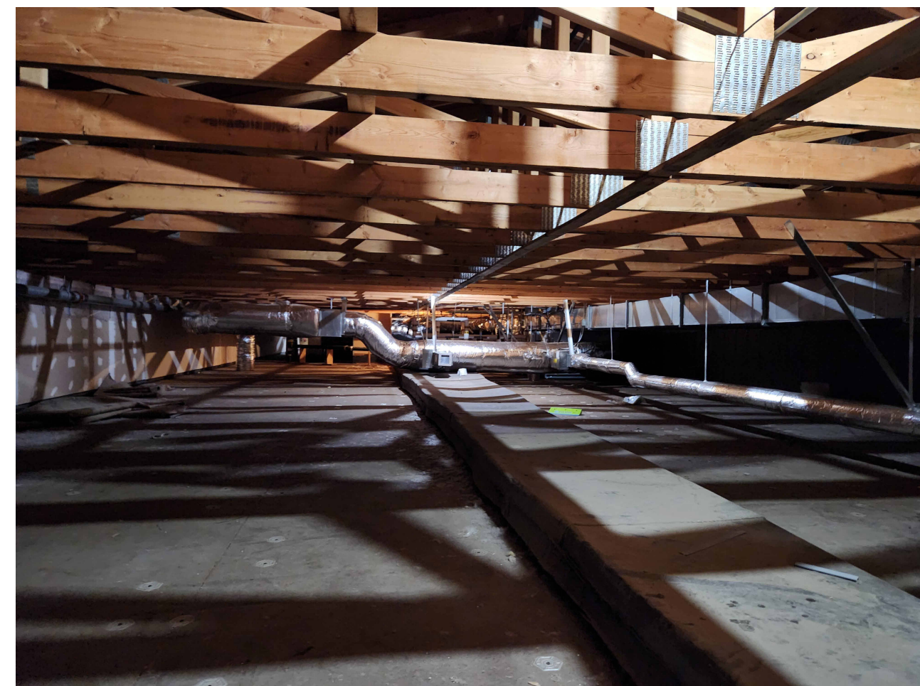
11 ATTIC - LOOKING BACK NORTHEAST
