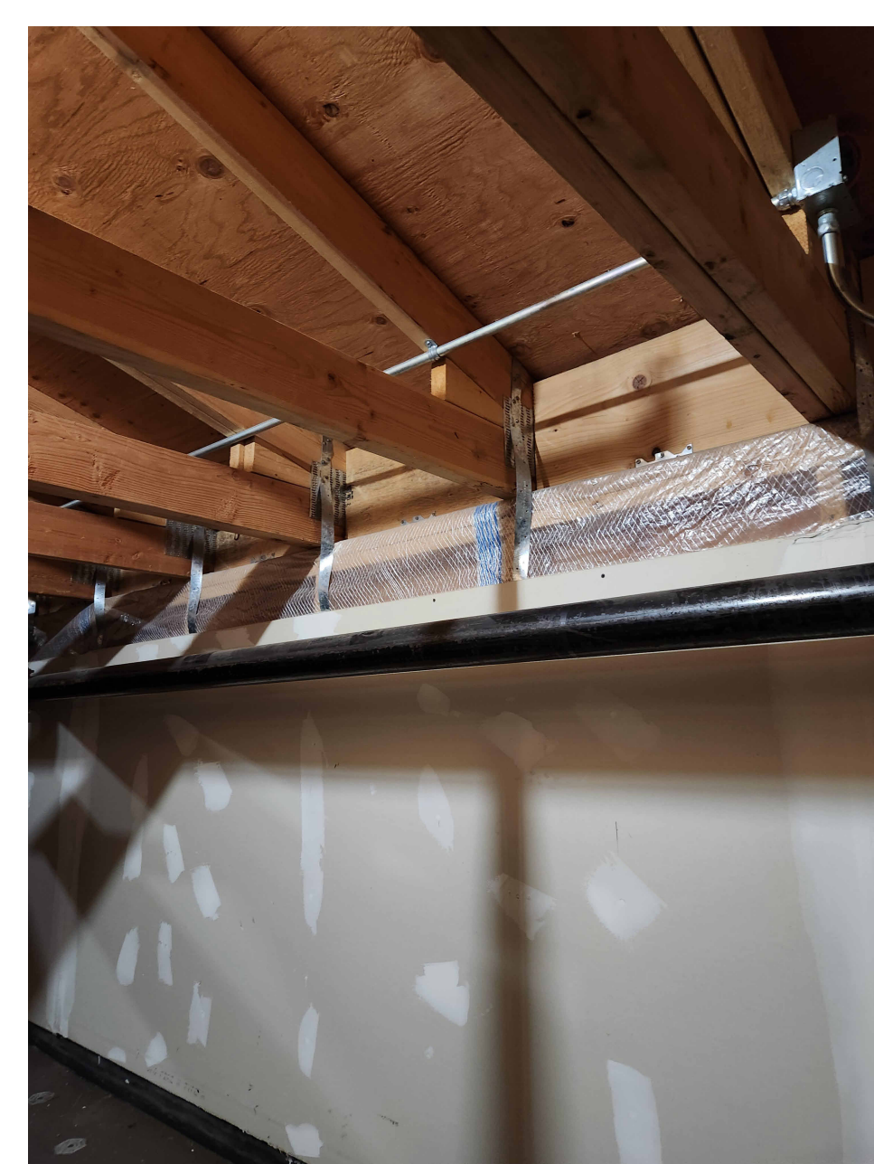
5 ATTIC SIDE WALL AND TRUSS EAVE
