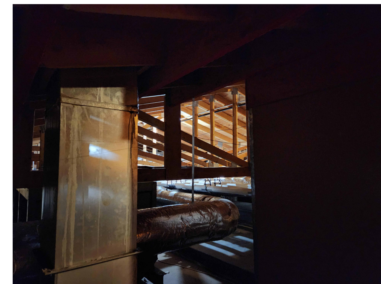
13 ATTIC - AREA OF HIGHER RAFTER FRAMING
