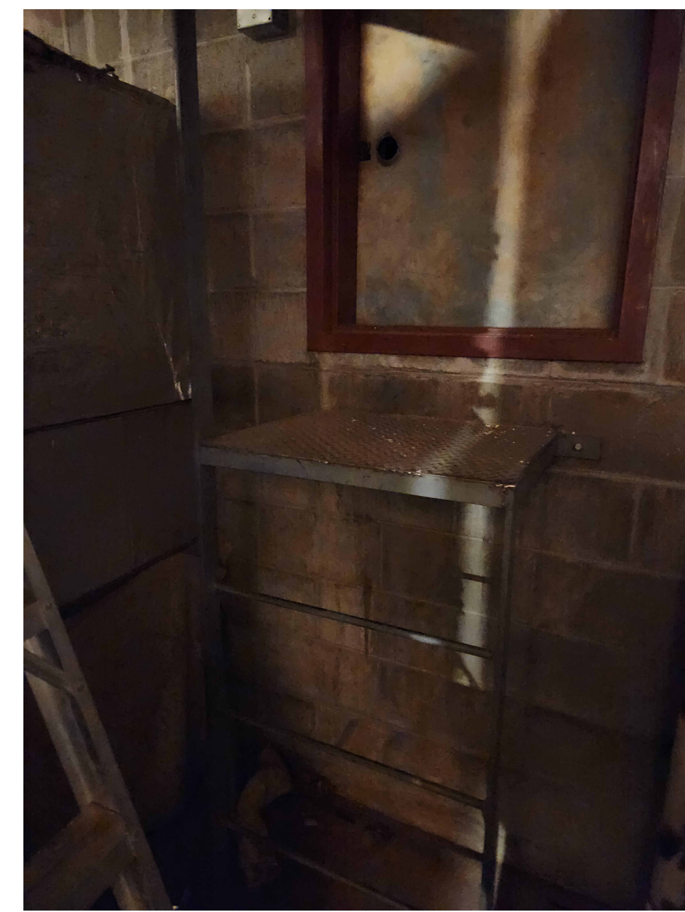
4 FAN ROOM - ATTIC ACCESS LADDER AND DOOR
