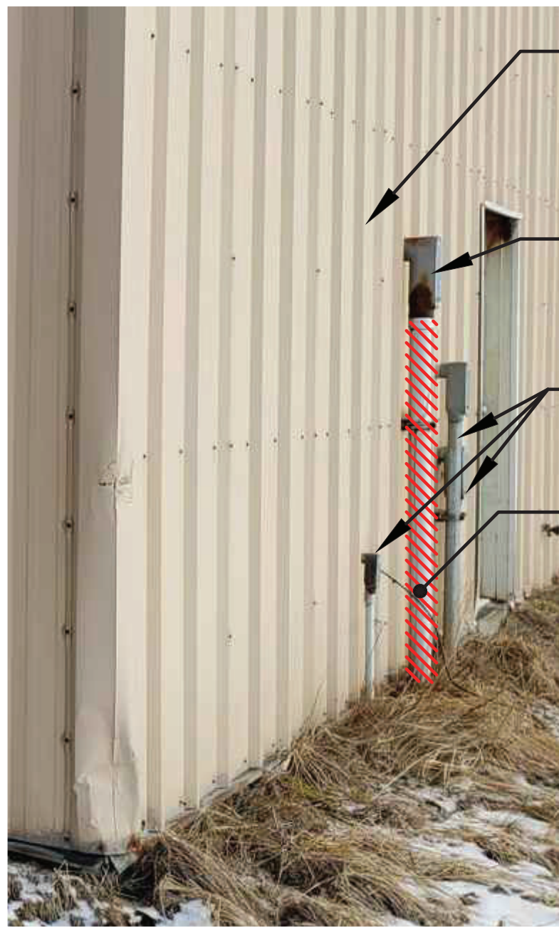
STORAGE COMPOUND 480V 3Ø SERVICE DEMOLITION
