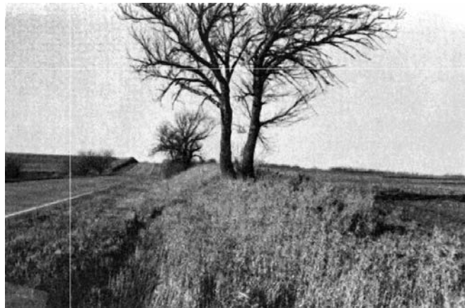
Figure 1160-4 Rural Roadside Hazard Rating of 4
