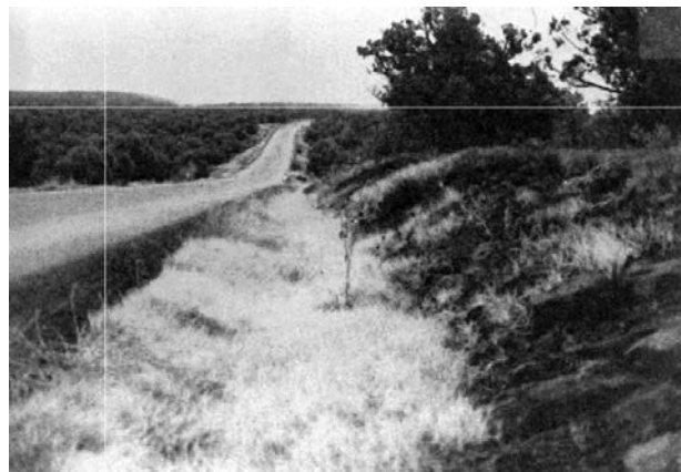
Figure 1160-3 Rural Roadside Hazard Rating of 3
