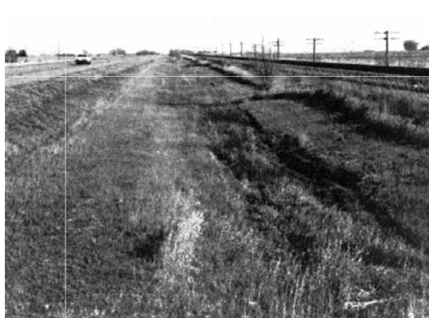
Figure 1160-2 Rural Roadside Hazard Rating of 2
