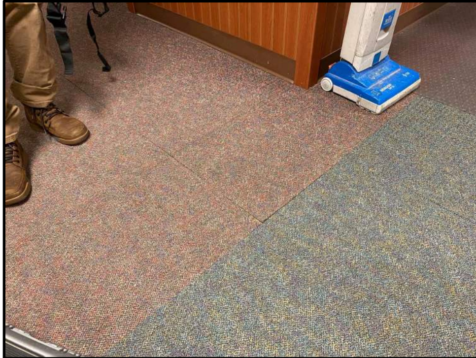
Photo 4: McKinley Hallway with multiple carpet types over green 9"x9" green tiles with black mastic containing greater than 1% asbestos as shown in Photo 1.
