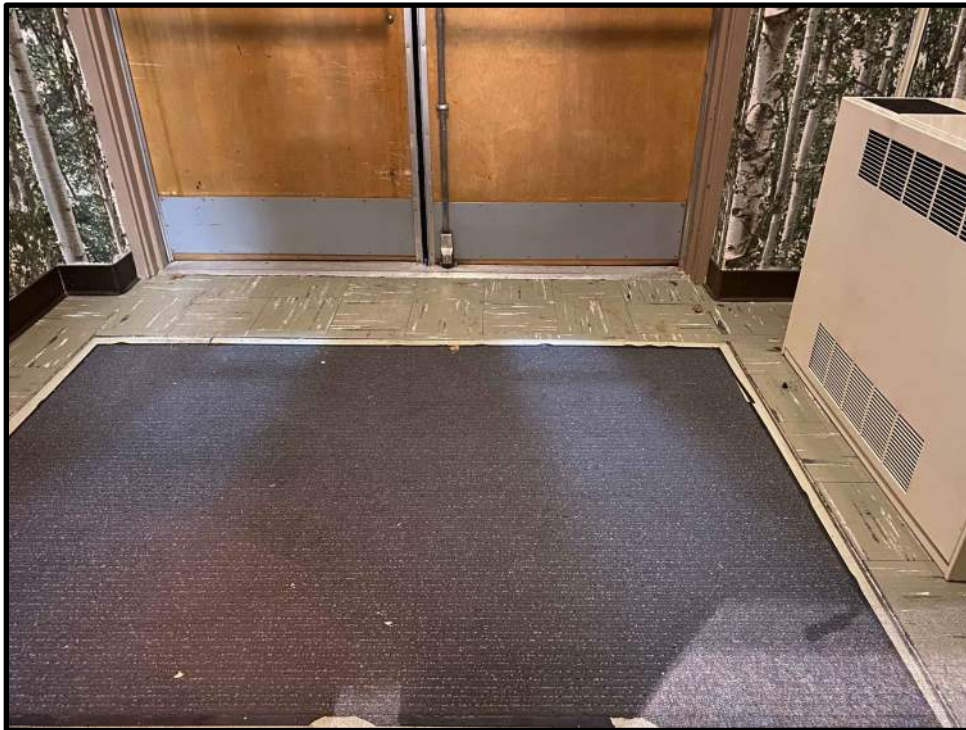
Photo 2: Multi-colored floor tiles with black mastic containing less than 1% asbestos in entryway at end of McKinley Hall
