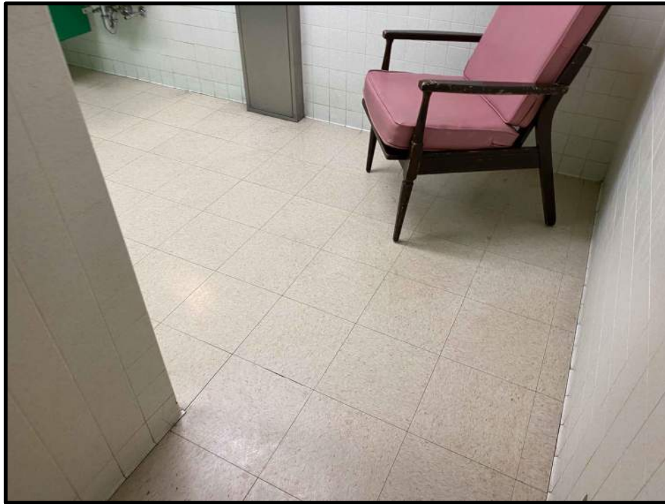
Photo 3: 12"x12" vinyl tiles in the men's locker room with black mastic containing less than 1% asbestos.
