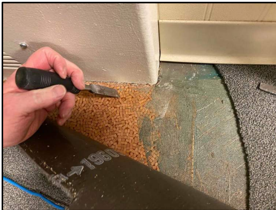
Photo 5: Location of Sample 25. Vinyl flooring under self-adhesive carpet in the conference room. Many variations and colors of vinyl were observed under carpeting throughout the building. Vinyl flooring and associated yellow mastic contain greater than 1% asbestos.
