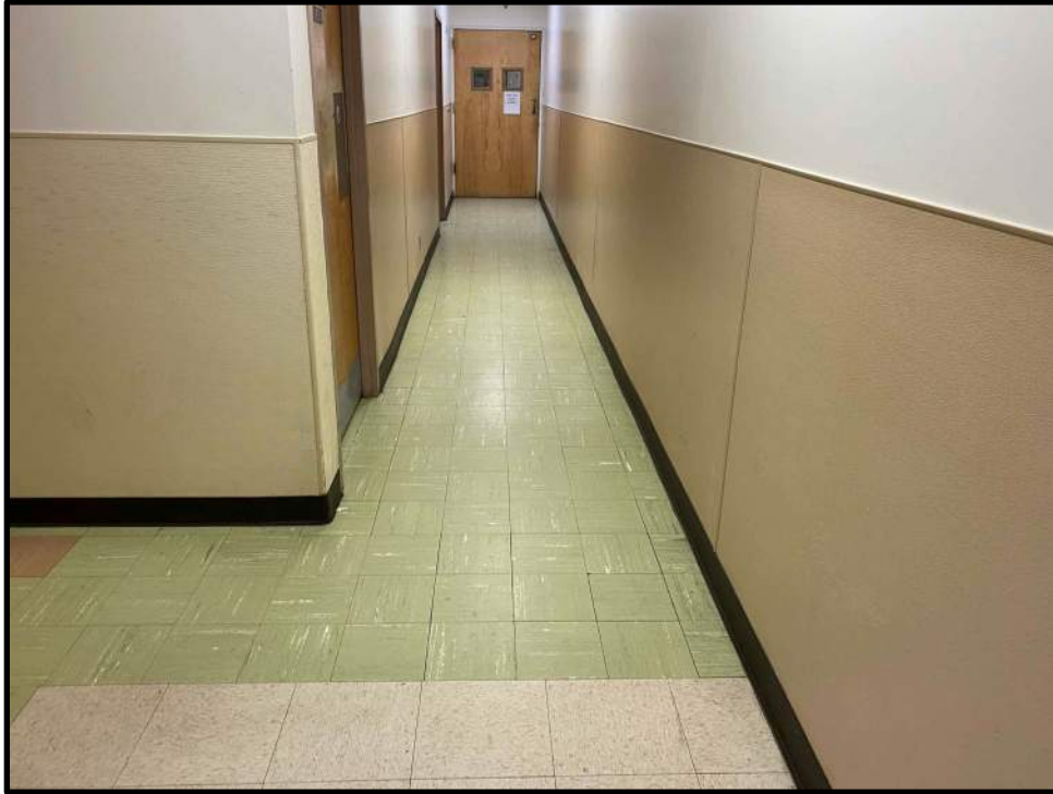
Photo 1: Green 9"x 9" tiles in Corridor 009. Both the tile and black mastic contain greater than 1% asbestos. These tiles and mastic extend into McKinley hallway and the adjoining solariums.
