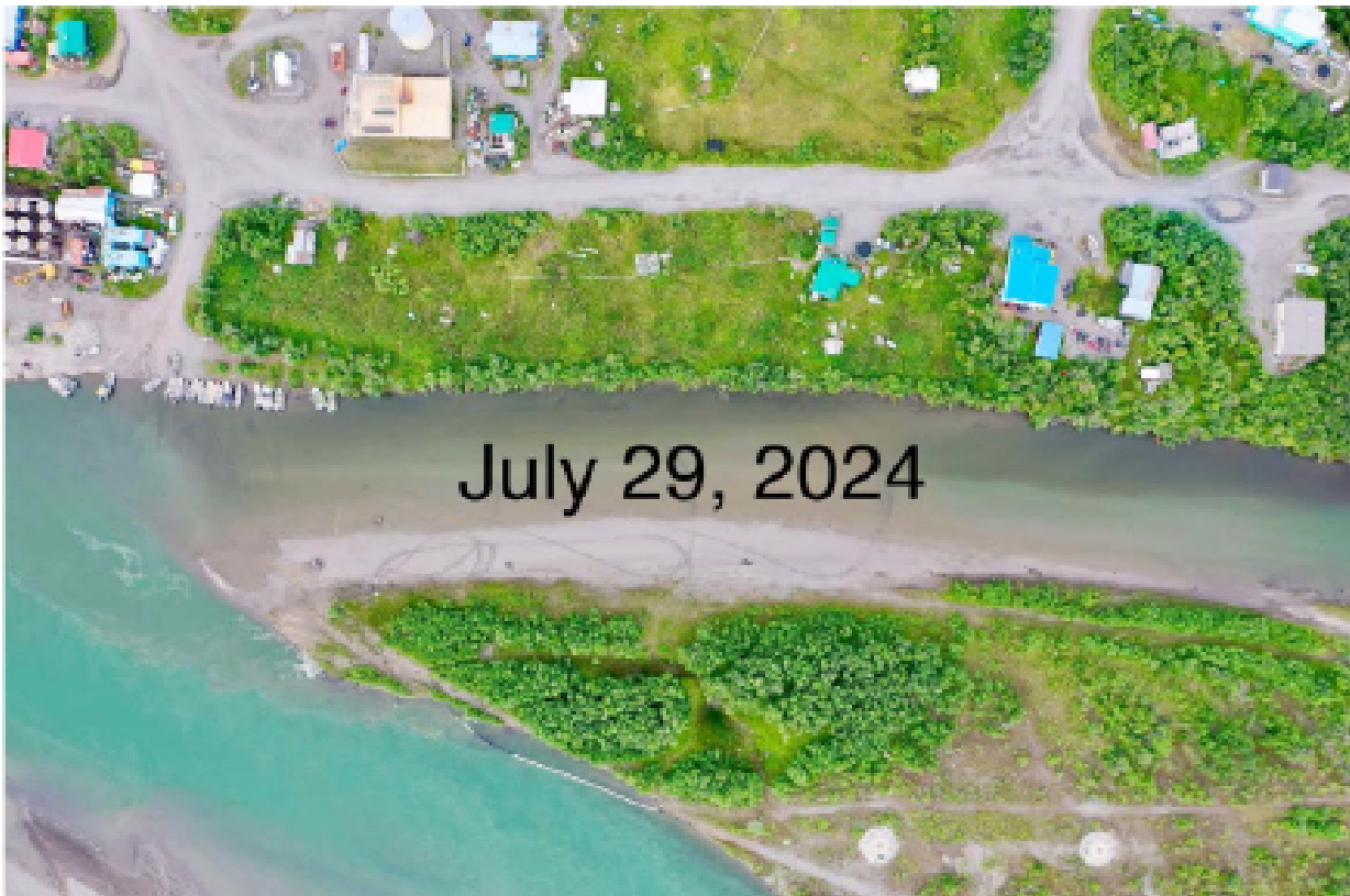
Figure 1: Approximately 125 feet of RWTL Floating in Noatak River
